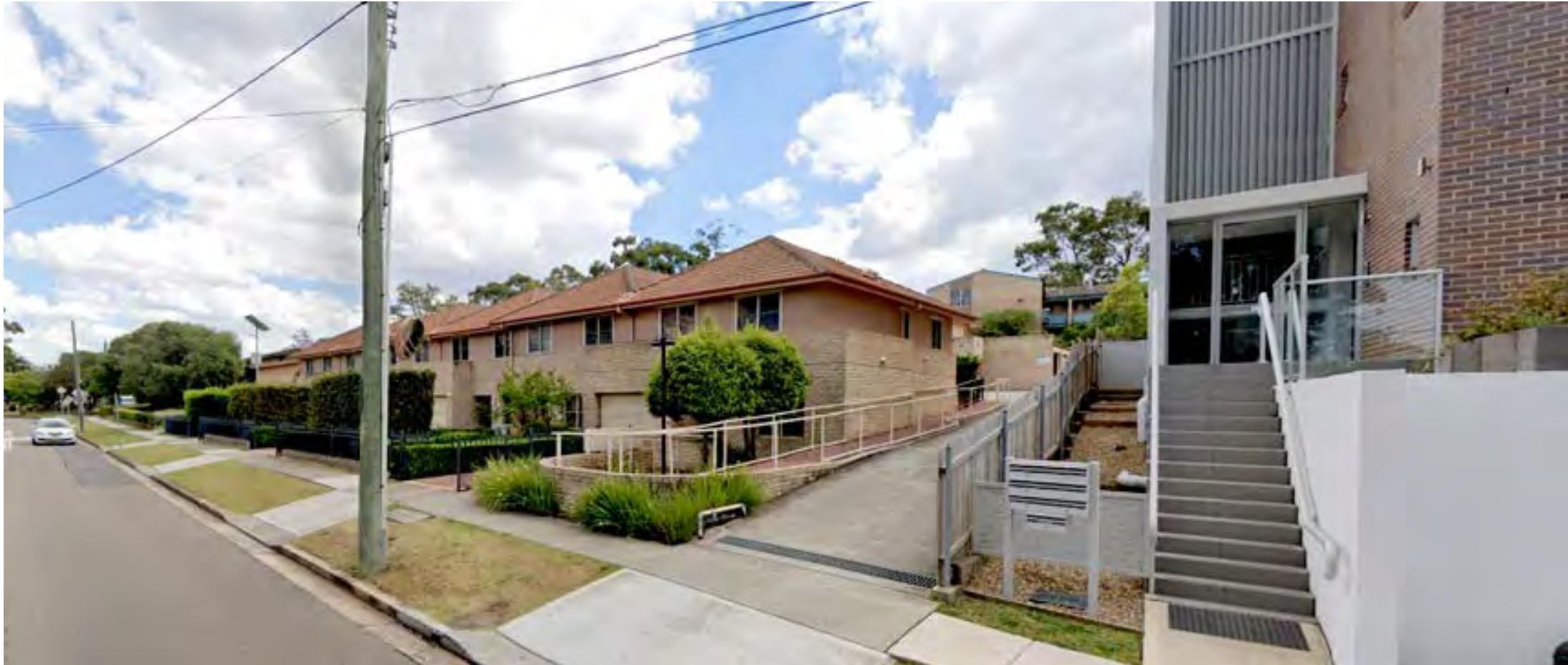
G. Manson Street existing street character
