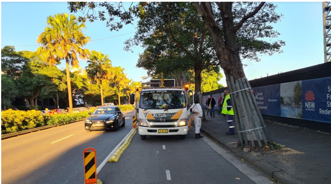
Figure 5 Temporary closure of Moore Park Road pop-up cycleway post event
