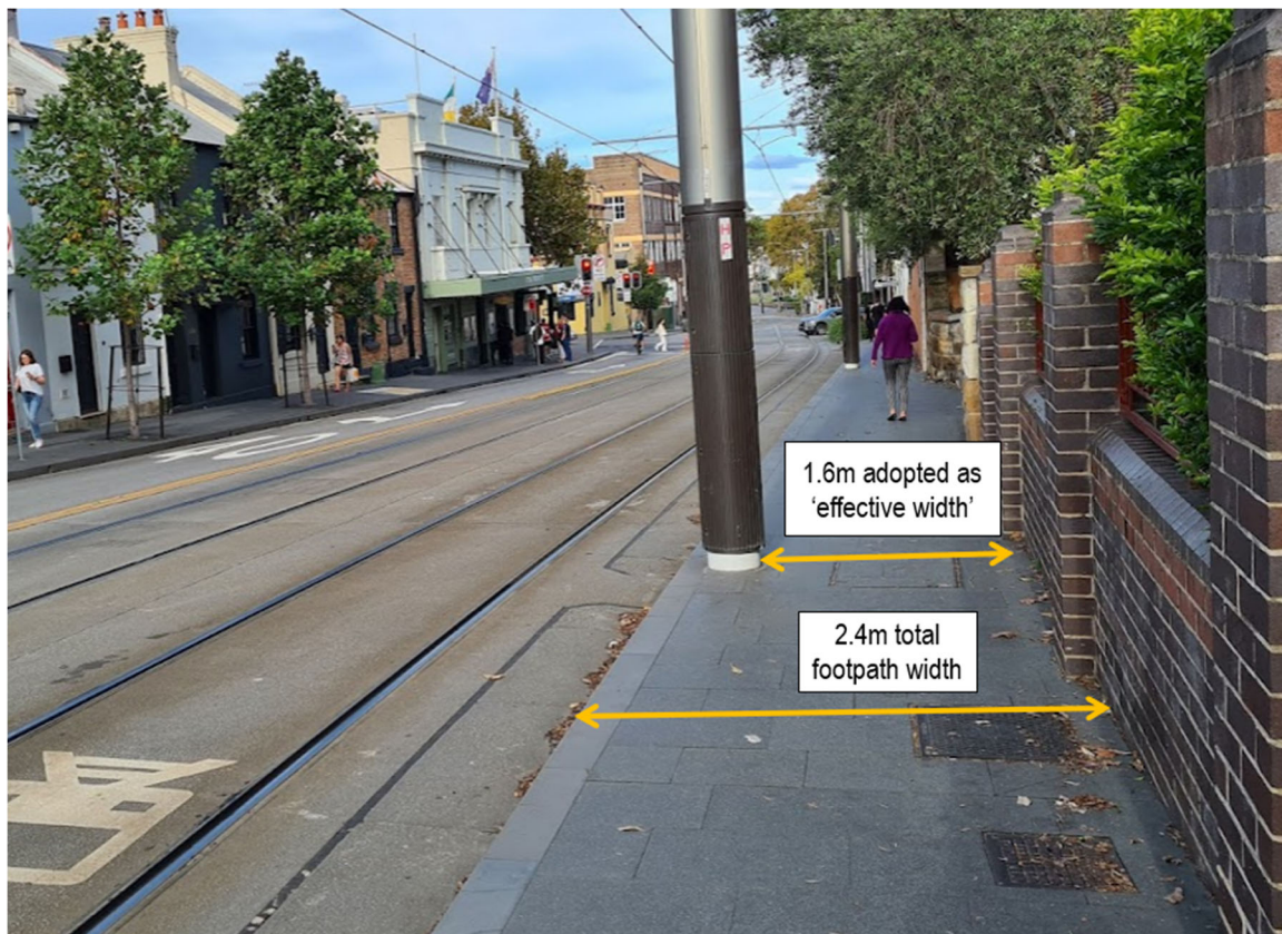
Figure 3 Example footpath width calculation on Devonshire Street
