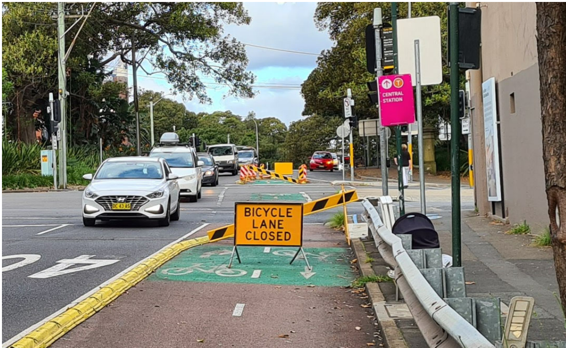
Figure 4 Temporary closure of Fitzroy Street pop-up cycleway post event
