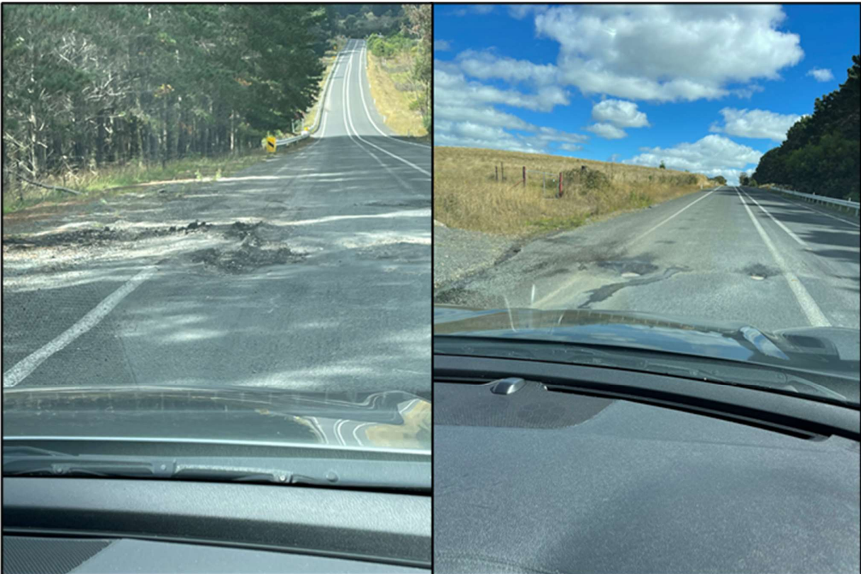
Figure 2.1: Red Hills Road Degradation
