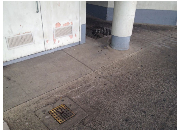
Figure 4.23: Example of subsurface services on the western side of the Harbourside Shopping Centre.
