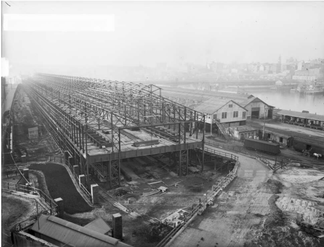
Figure 4.8: Framework of Darling Harbour Sheds construction (1920) Source: NLA PIC P860/325
