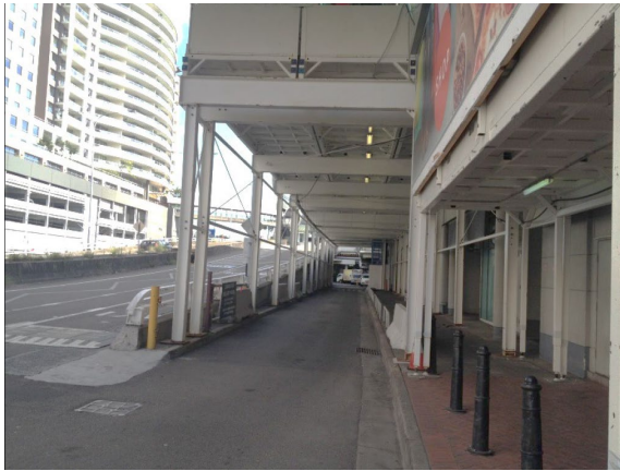
Figure 4.22: Loading dock entrance on western side of Harbourside, Darling Drive to the left.
