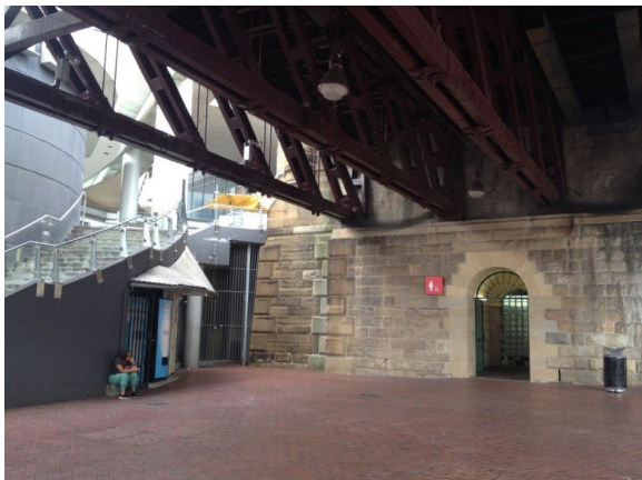
Figure 4.20: Northern boundary of Harbourside & sandstone foundation of Pyrmont Bridge, showing gated entrance to loading dock on northwestern side of Harbourside.
