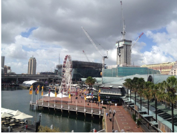
Figure 4.16: Eastern boundary of the Harbourside site showing interface with public promenade on the waterfront.
