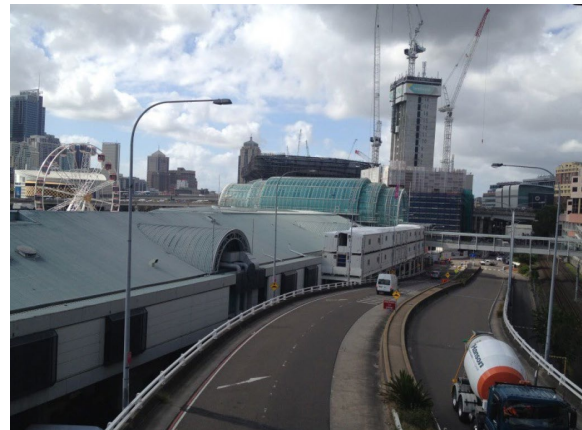
Figure 4.15: Western boundary of the study area facing south. Darling Drive runs along the western boundary. The light rail line to the west of Darling Drive follows a route of the original Darling Harbour Goods line.
