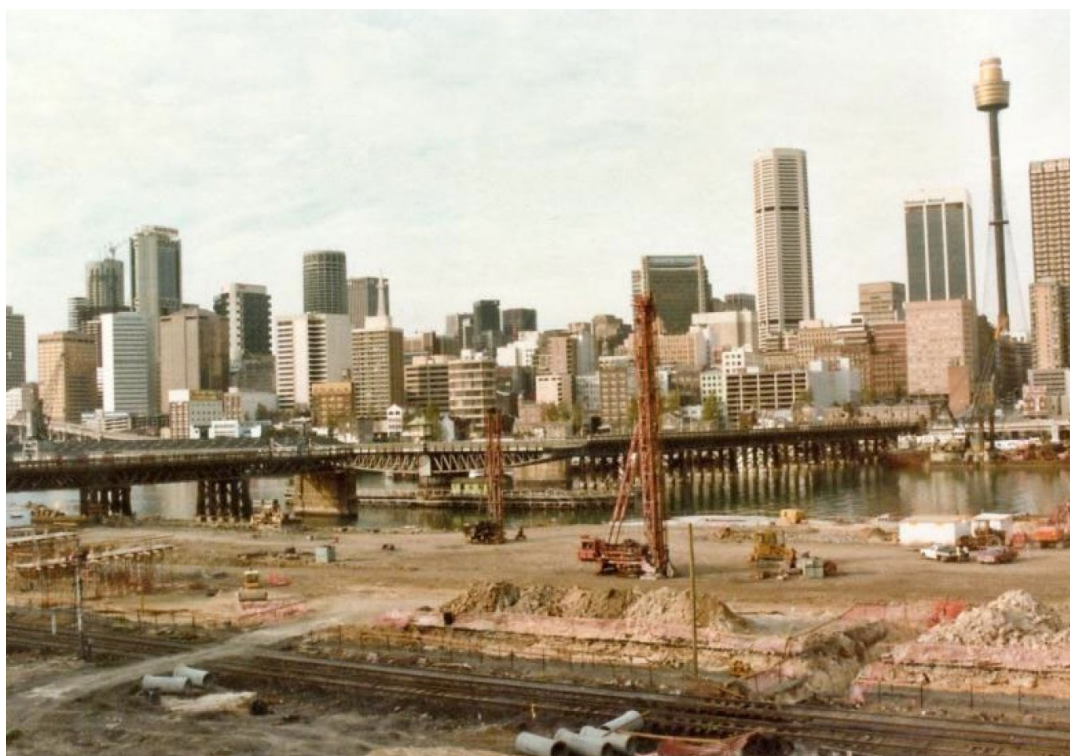
Figure 4.10: Construction of the Harbourside Centre (1980s) Source: Sydney Harbour Foreshore Authority
