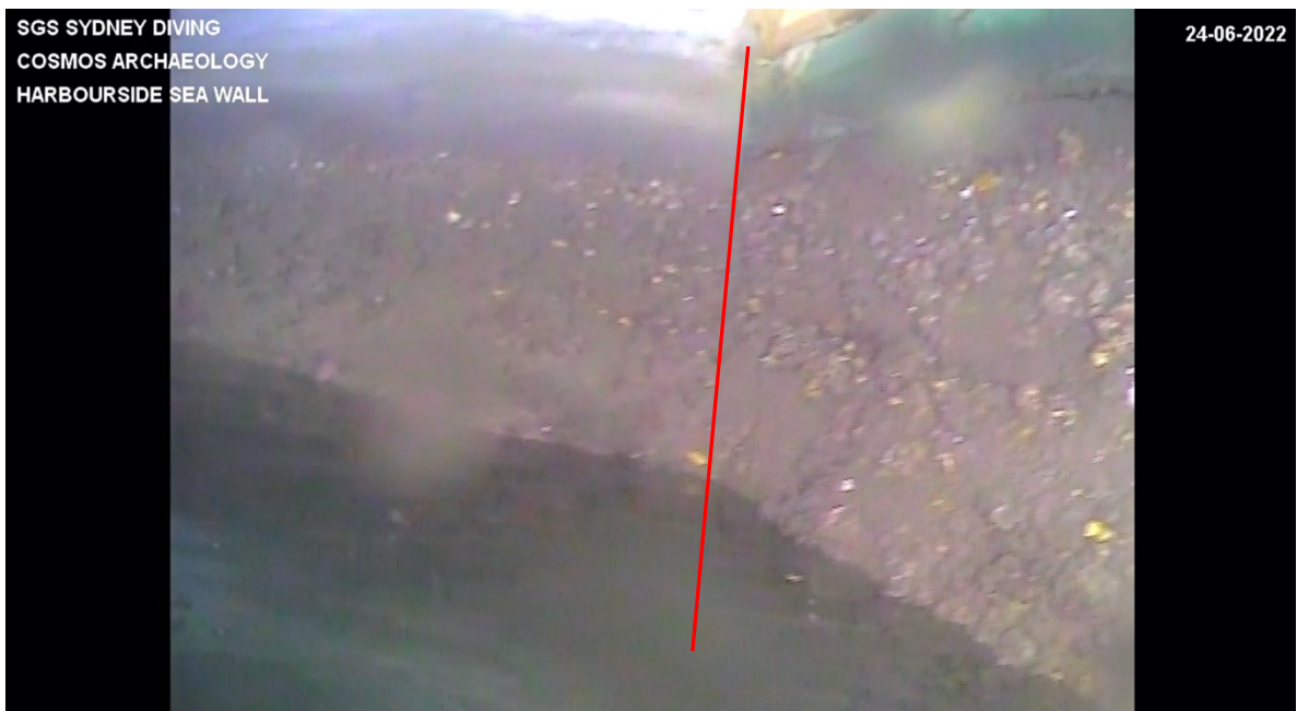
Figure 20: Junction of modern concrete seawall to the left of image and stone seawall to the right. (Image from 220624_Stone seawall dilapidation_S_walkway, 01:48).
