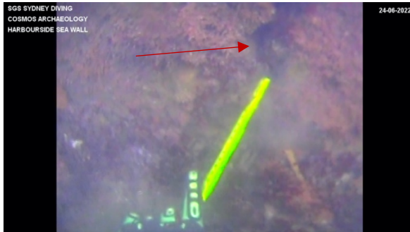
Figure 11: Example of gaps between blocks indicating mortar loss. (Image 220624_Stone seawall dilapidation_1, 04:18)
