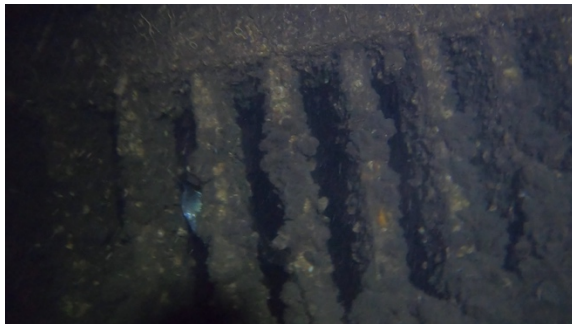
Figure 27: Example of growth build-up on intake gates. (Image 220624_Intake conduit, 03:34).
