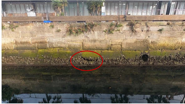
Figure 9: Example of mortar loss above water. (Image 220624 Harbourside stone wall above water_linear, 01:41).
