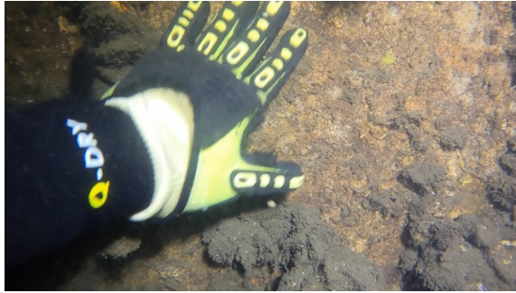
Figure 25: External concrete wall of intake entrance. (Image 220624_Intake conduit, 00:11).
