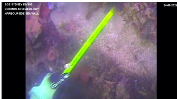
Figure 15: Section of undermining at base of stone wall 39 m along survey line. (Image 220624_Stone seawall dilapidation_3, 00:03)
