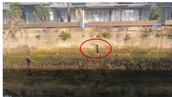
Figure 8: Some evidence of a repair using bricks. (Image 220624 Harbourside stone wall above water_linear, 01:28).
