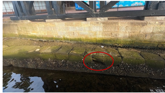
Figure 6: Stone seawall underneath the Pymont Bridge. Note mortar loss. (Image 220624 Harbourside stone wall above water_linear, 00:13).
