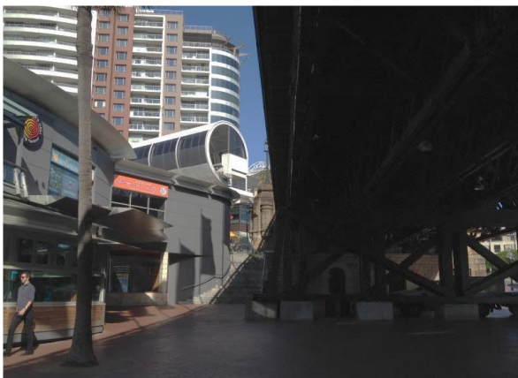
Figure 4.5: Interface between Harbourside (left) and Pyrmont Bridge (right), view facing west. the former Monorail Station is visible in the centre of the image.
