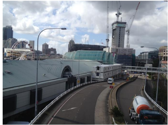
Figure 4.2: Western boundary of the subject site, view facing south. The light rail line to the west of Darling Drive follows a route of the original Darling Harbour Goods Line.
