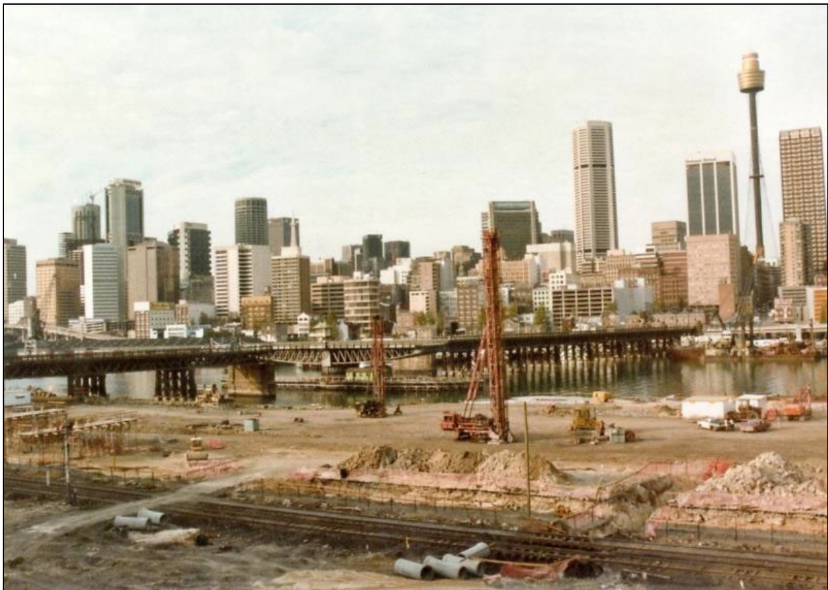
FIGURE 16: CONSTRUCTION OF HARBOURSIDE, 1980S. SOURCE: SYDNEY HARBOUR FORESHORE AUTHORITY, HTTP://WWW.SHFA.NSW.GOV.AU/SYDNEY-ABOUT-US-HERITAGE-ROLE-HERITAGE-AND-CONSERVATION-REGISTER.HTM&OBJECTID=173
