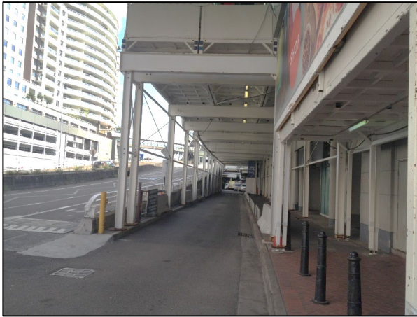
FIGURE 25: LOADING DOCK ENTRANCE ON WESTERN SIDE OF HARBOURSIDE. DARLING DRIVE RISES ON THE LEFT HAND SIDE OF THE IMAGE. TEMPORARY CONSTRUCTION SHEDS ARE INSTALLED ABOVE THE LOADING DOCK DRIVEWAY.
