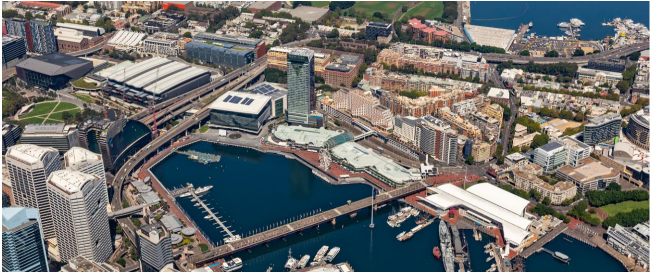
Figure 5 Aerial image of the existing development on the site
