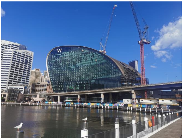
'The Ribbon' building (nearing completion)
