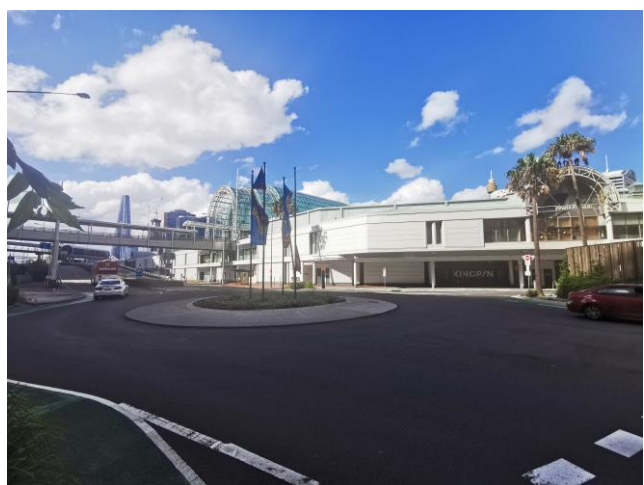
Rear of the site, facing Darling Drive
