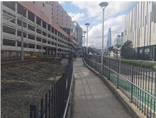
Inner West Light Rail tracks and Pyrmont station
