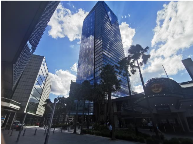
Sofitel Hotel tower
