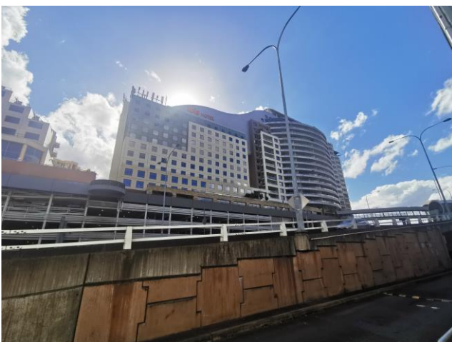
Ibis Hotel and 50 Murray Street apartments
