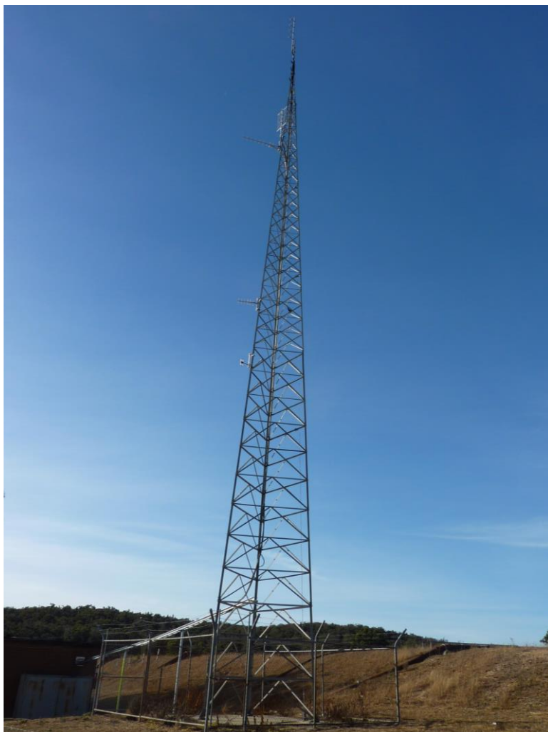
Figure 4 telecommunications tower and dam embankment
