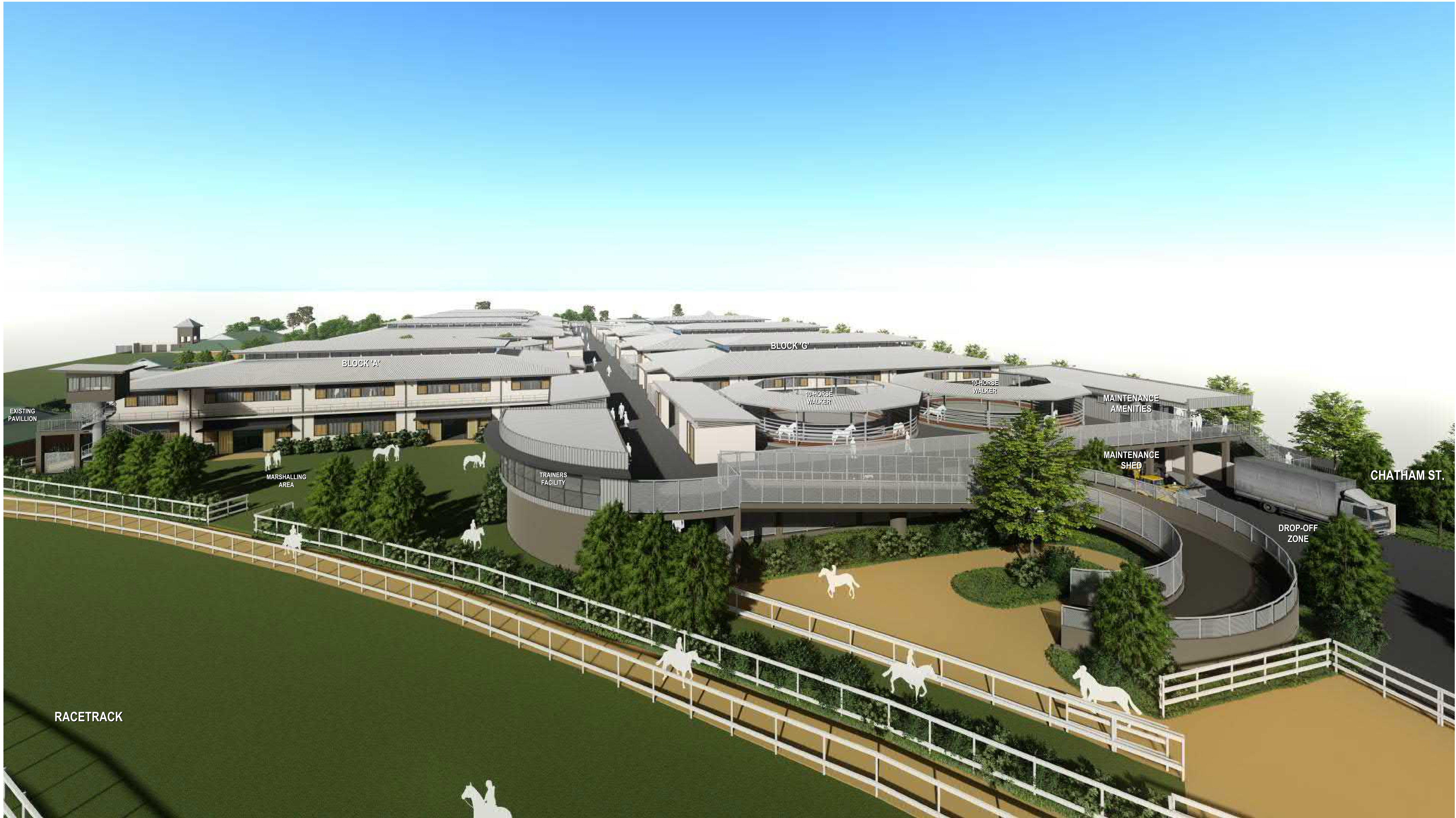
VIEW FROM NORTH
