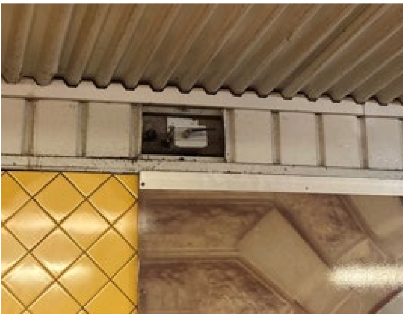
Figure 7 – Existing vibration monitors within Central Station.
