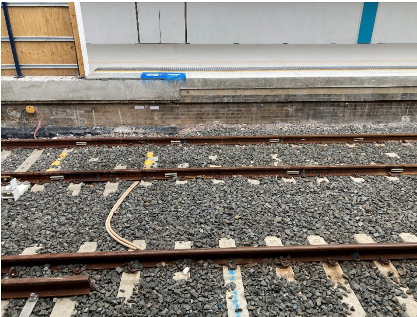
Figure 6 – Existing track monitors adjacent to platform.
