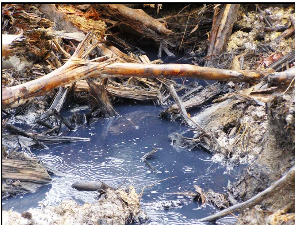
Plate 3: Tannin generation from recently felled and partially mulched vegetation in an area subject to localised inundation. Mulched vegetation should be progressively moved to prepared stockpiles to manage tannin impacted water.
