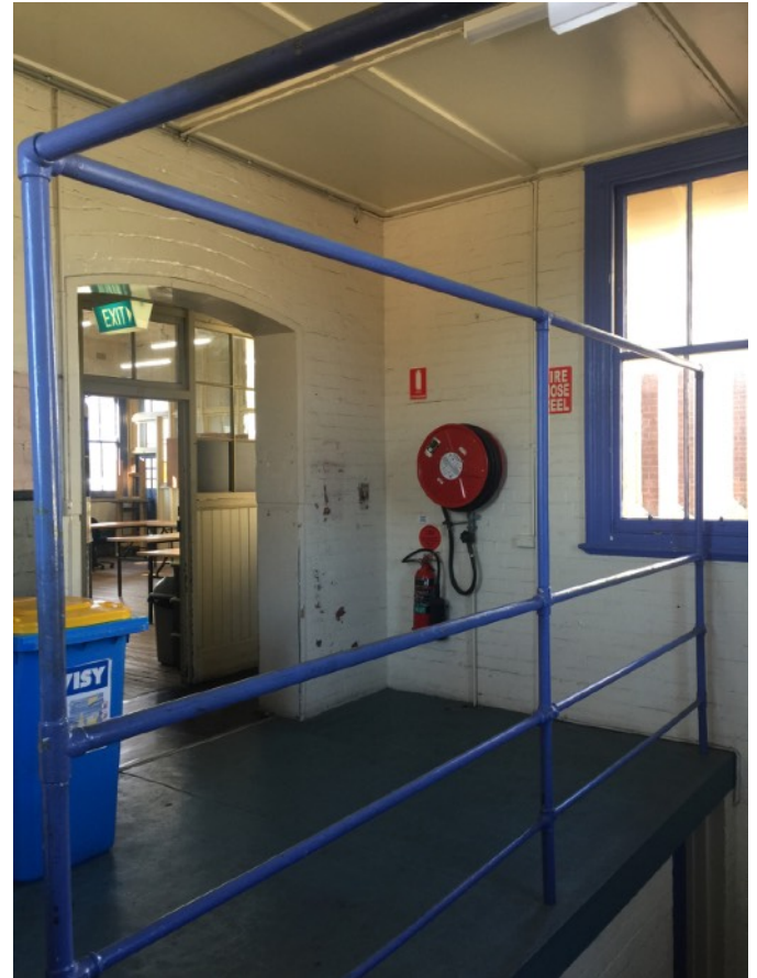
6. View of the non compliant and later pipe hand rail in the lobby. It is proposed to replace the non compliant handrail with a compliant metal handrail.
