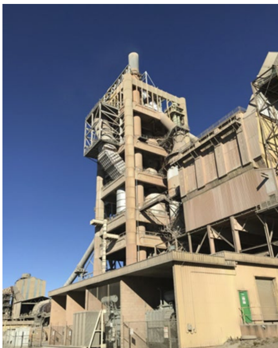
EPA 2 – No.6 Kiln Stack
