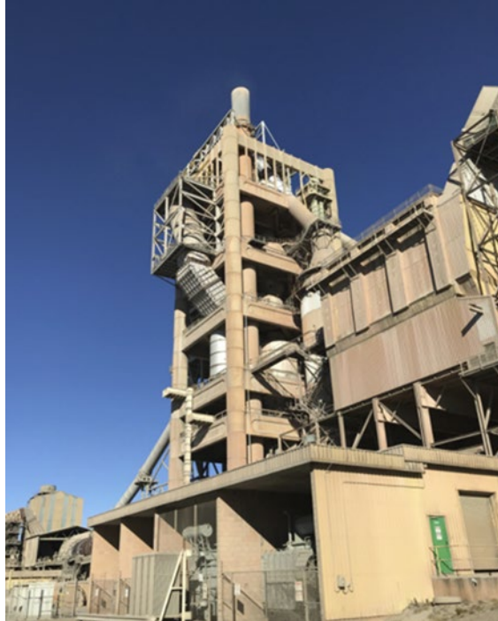
EPA 2 – No.6 Kiln Stack
