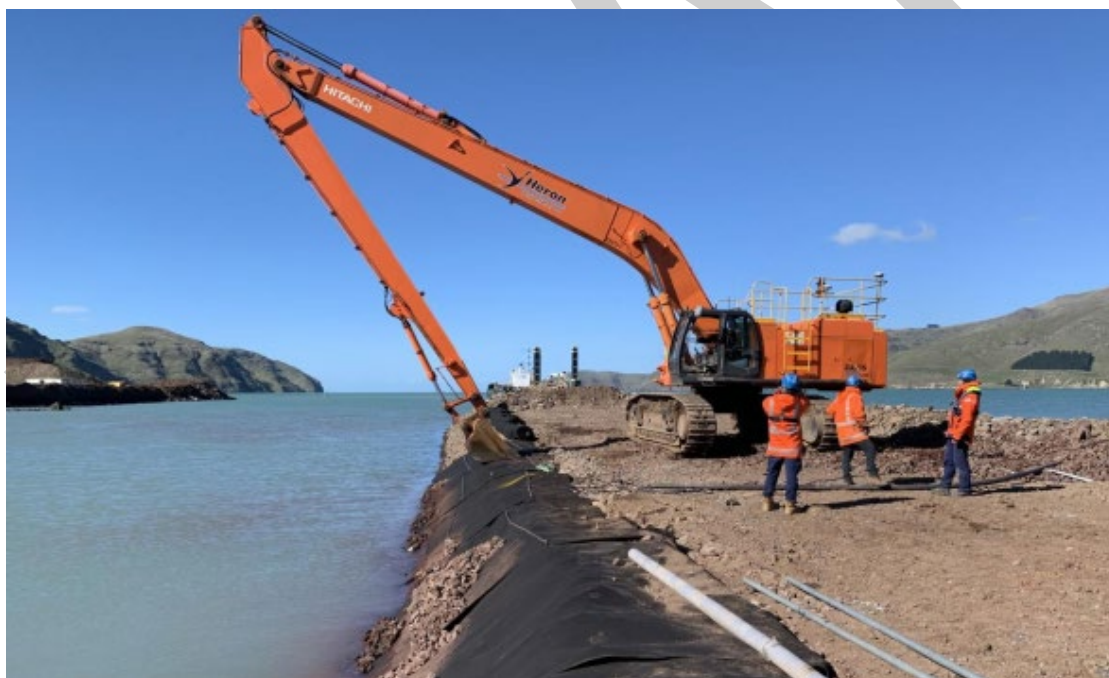
Figure 10.8 Longreach assisting in geotextile installation
