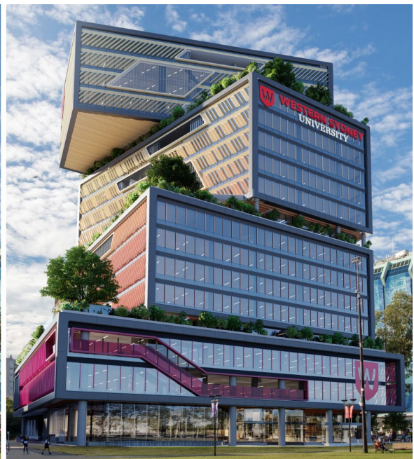
Picture 2 Modified Signage Zone
