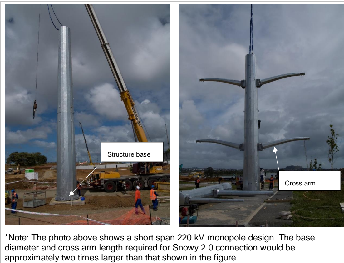
Figure 1: Typical steel monopole for a 220 kV connection.
