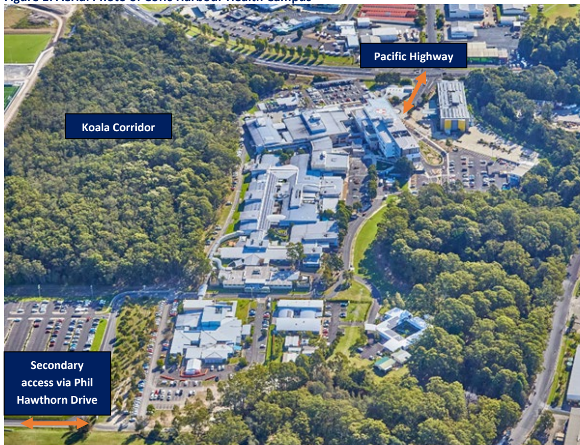
Figure 1: Aerial Photo of Coffs Harbour Health Campus
