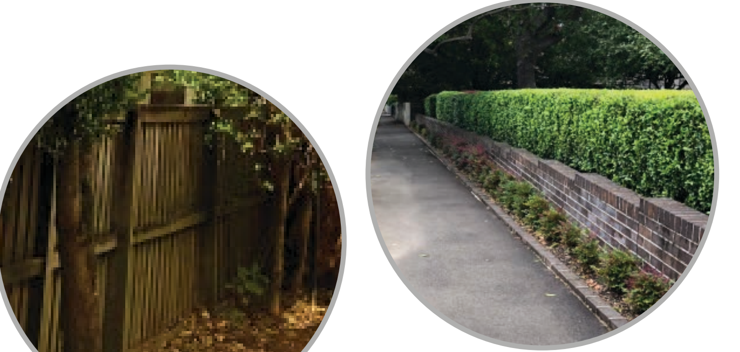
Existing photo of timber boundary fence north-south between new SWELL building and 39 Bancroft Avenue. Proposed new fence to be replaced with slightly modify detail including 3 rail, lapped and capped with metal posts.
