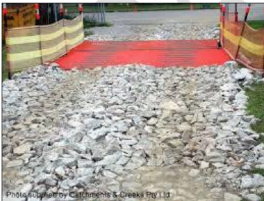
Figure 6.2 Gravel haul road to be installed at MBD Site Compound and Emplacement Cell Construction Sites
