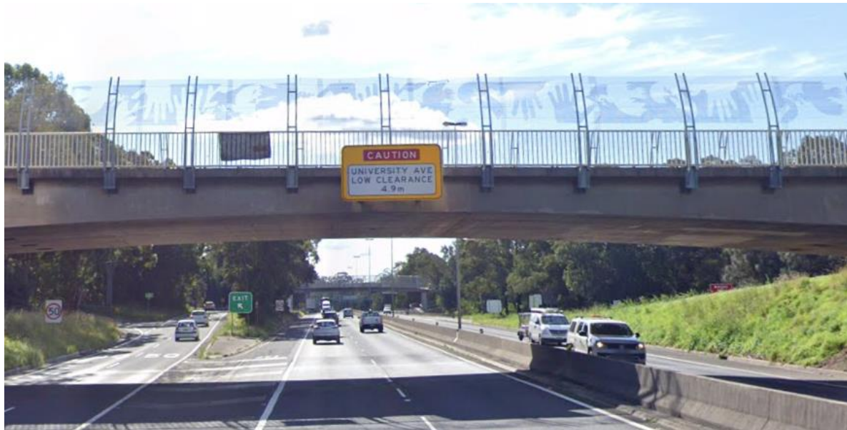
Figure 2.6: Height restriction - University Avenue footbridge, Gwynneville
