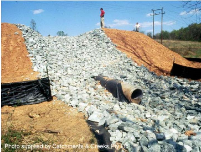
Figure 32 - Sediment Basin Spillway
