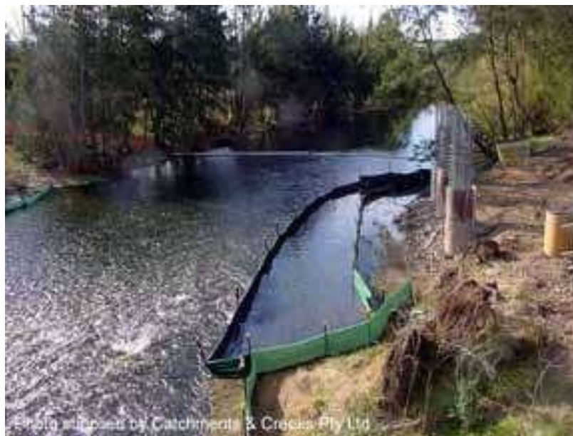
Figure 12 - Instream isolation barrier
