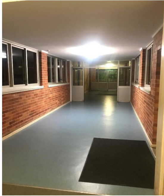
Photograph 19: B00B, BR1023, floor below vinyl sheeting, possible vinyl tile containing asbestos, limited access for inspection.
