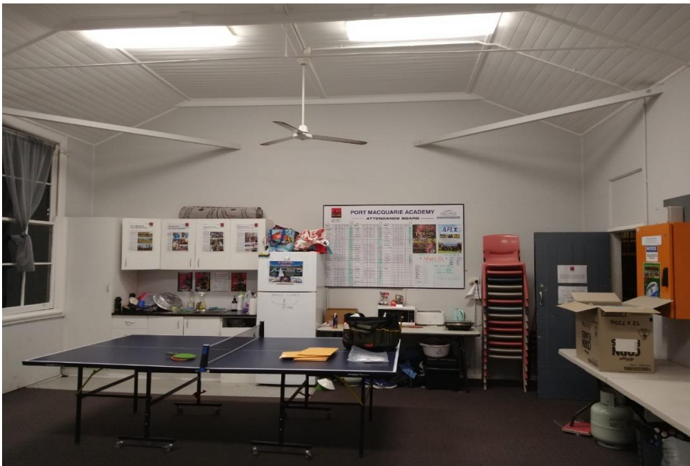
Photograph 2: B00S, SR0002, walls throughout, undercoat paints, positive for lead.
