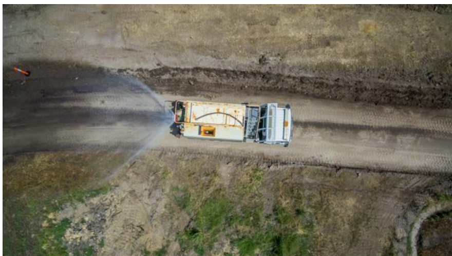
Figure 15 - Water cart application of soil binder
