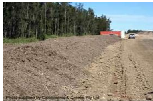
Figure 24 - Mulch berm
