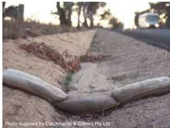
Figure 8 - Sand bag check dams
