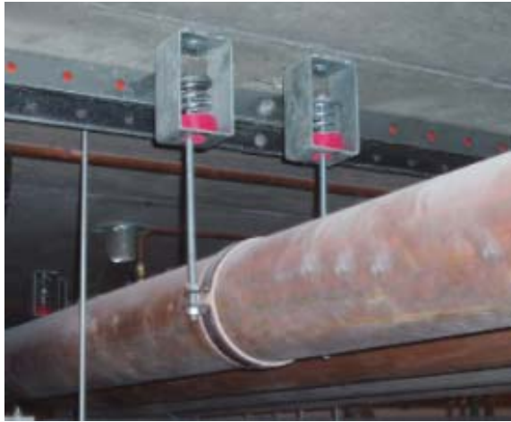
Figure 3. Embelton Isolation Hangers
