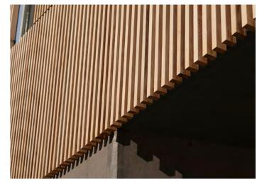
**06** Timber battens on aluminum framing
