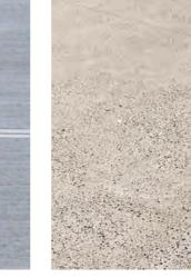
02 Exposed aggregate concrete paving
