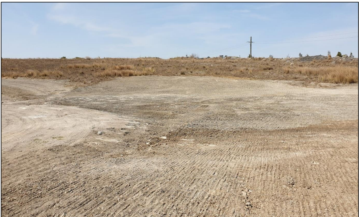
Photo 3 Rehabilitation of Gas Well Site GW14/3 (Prior to Seeding)
