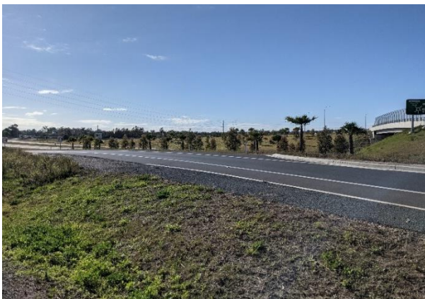
Photo 36: Maclean Interchange – landscaping and signage
