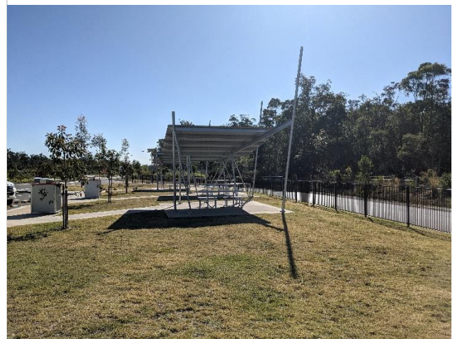
Photo 29: Pine Brush rest area
