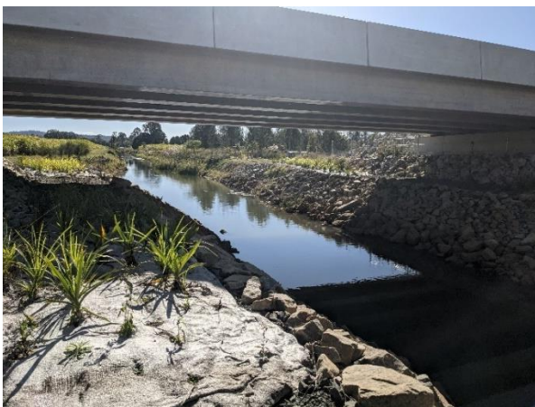
Photo 34: Emu underpass – Crackers Drain
