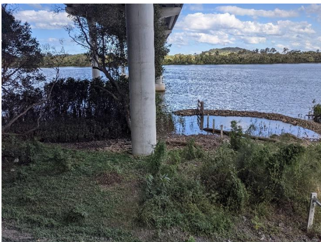
Photo 30: Rehabilitated mangroves with seed capture structure, Richmond River – Backchannel Road
