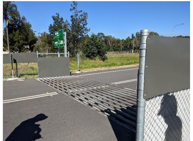
Photo 23: Koala grid on local road – Coolgardie interchange
