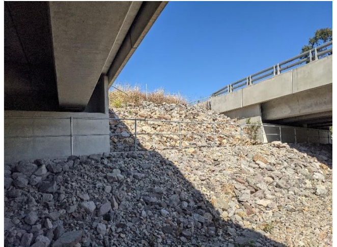
Photo 2: Corindi Creek crossing – new fence being planned for.
