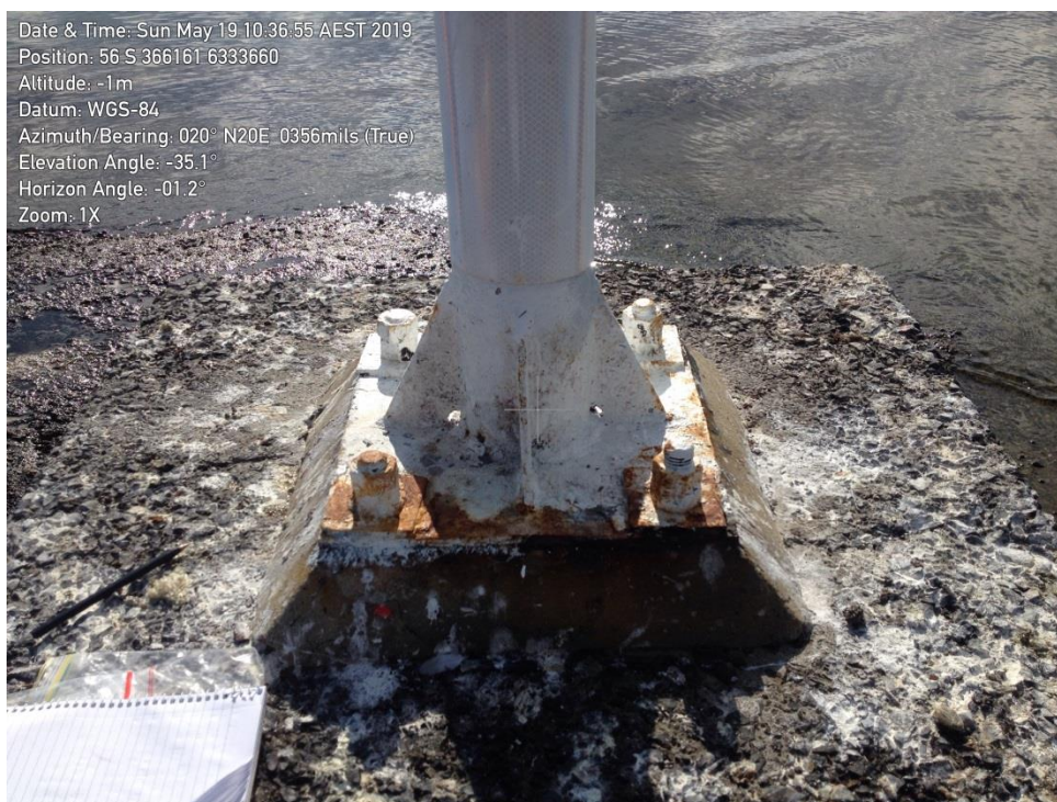
Photo 3. Current condition of the marker fixing to the concrete block
