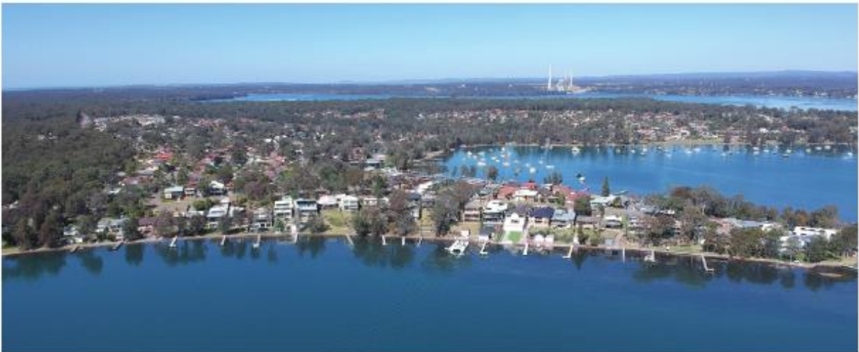
Figure 4: Aerial Photography of the Built Features along the Foreshore at Summerland Point
