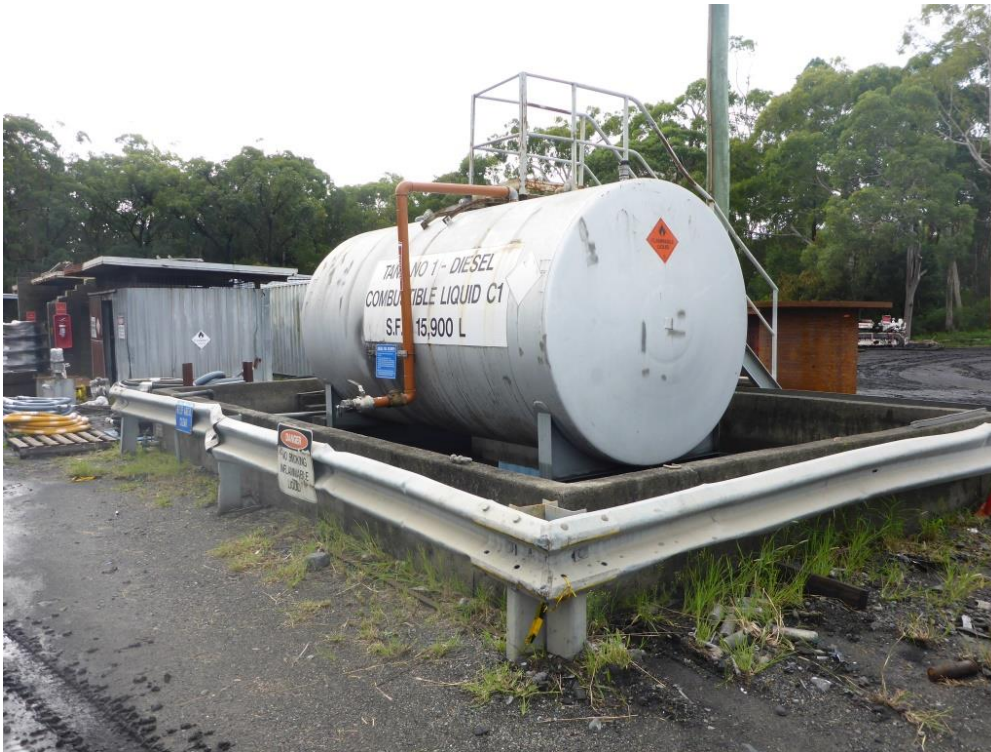
Photo 5 Diesel Tank stored within Bund
