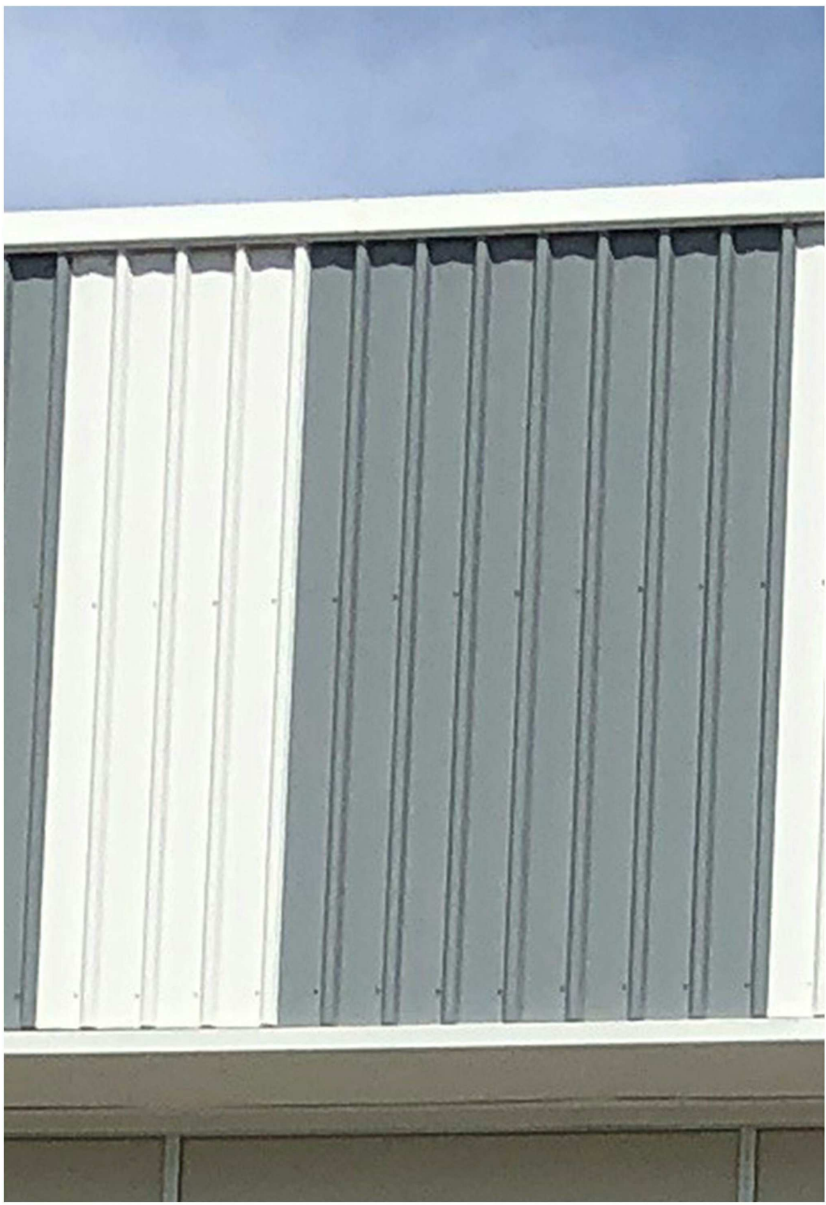
PROFILED METAL CLADDING
