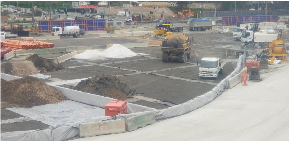
Figure 6 Example of bundled containment with drainage lines
