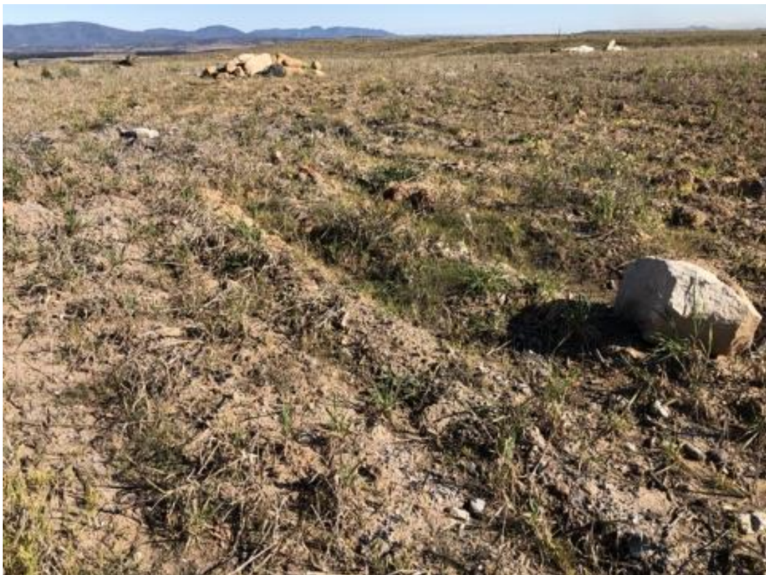
Plate 8 - Surface preparation with deep ripping and rock piles for native animal habitat.
