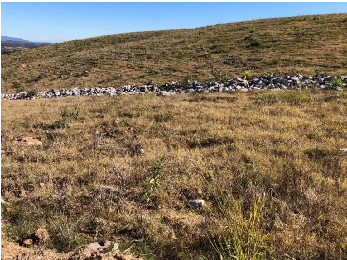
Plate 6 - Geomorphic landform with keyed in drainage line, surface deep ripped on contour to increase infiltration and reduce runoff. Note young trees establishing.
