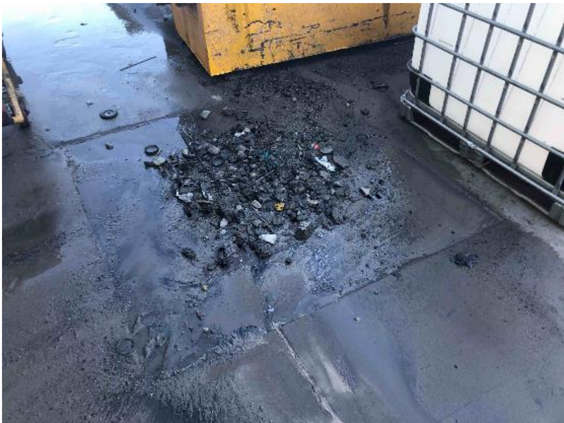
Plate 10 - Sediment build up over drains on workshop apron
