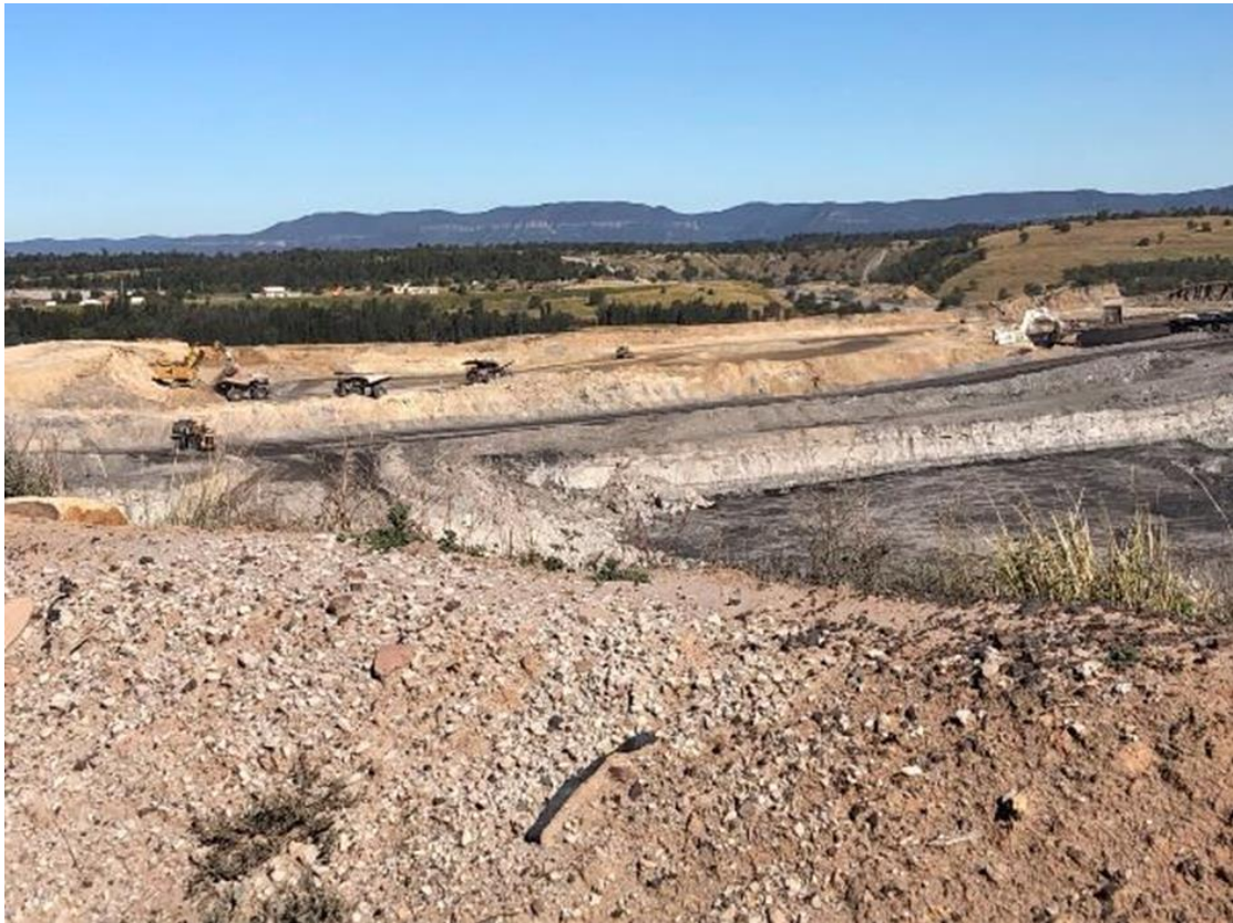
Plate 9 - Soil and overburden stripping in progress to the south of main pit.
