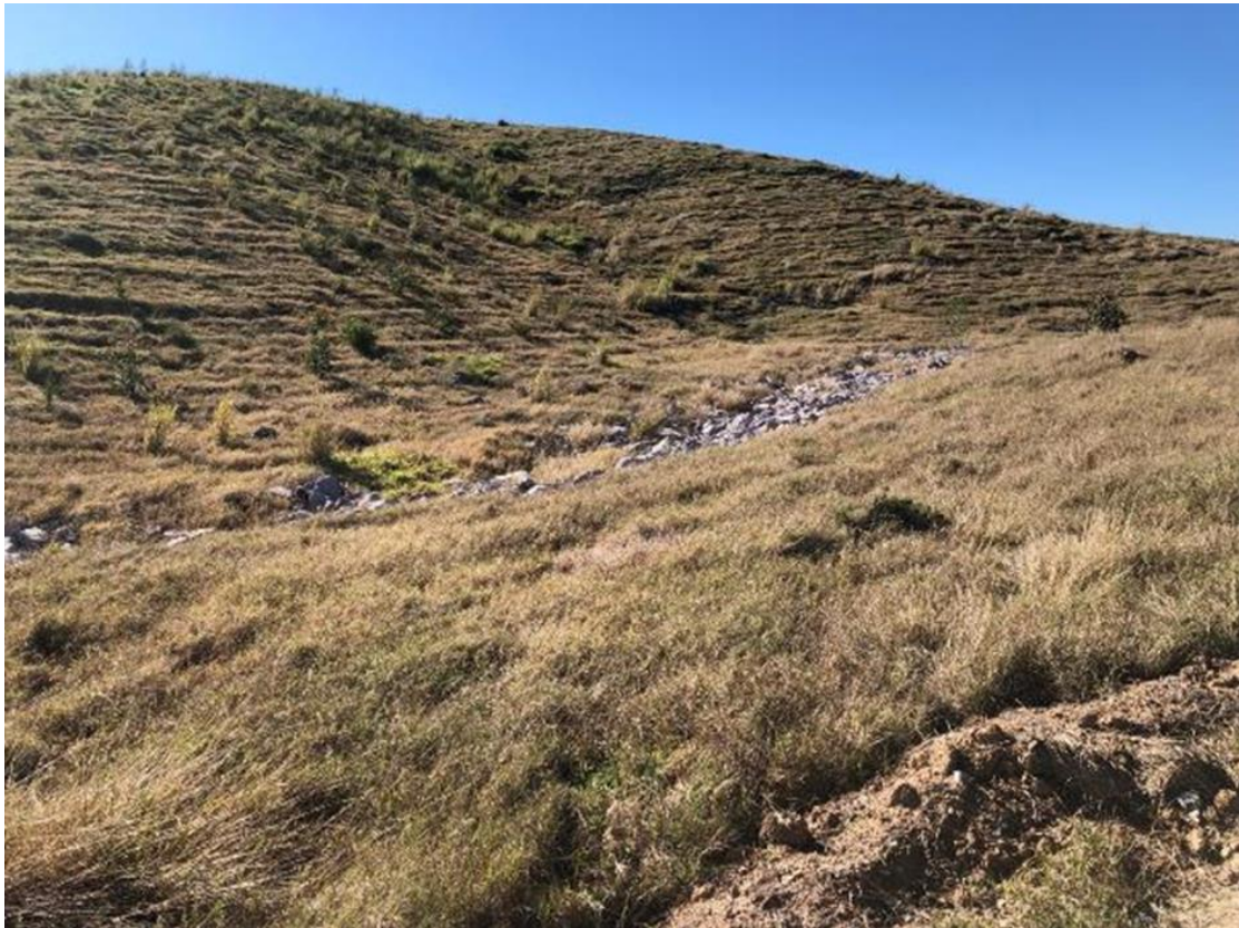
Plate 3 - Geomorphic designed landform with rock-lined drainage line.
