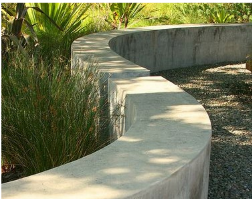
Concrete retaining walls
