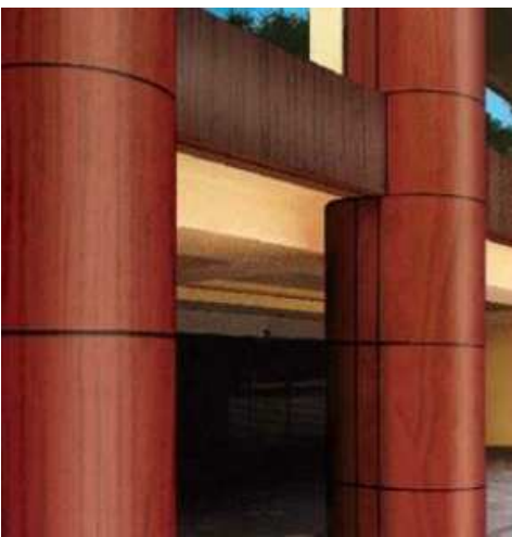
MC01 - ALUMINIUM CLADDING AROUND STEEL COLUMNS
