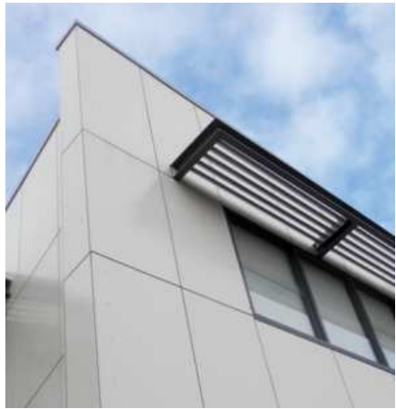
CFC01 - COMPRESSED FIBRE CEMENT
