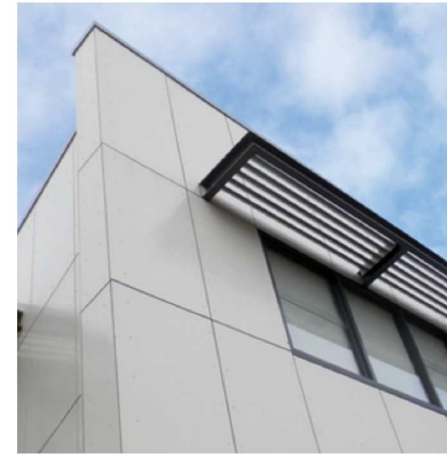
CFC01 - COMPRESSED FIBRE CEMENT
