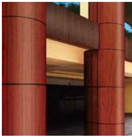
MC01 - ALUMINIUM CLADDING AROUND STEEL COLUMNS
