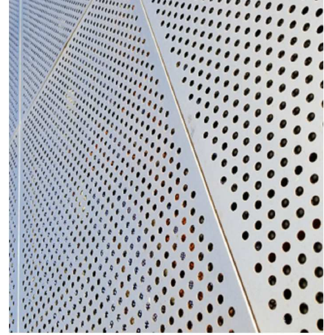
ALUMINIUM CLADDING AROUND COLUMNS AND LV03 SUNHOODS
