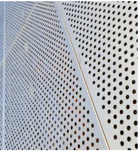
SCN02 - PERFORATED ALUMINIUM SCREEN COLOUR TBC
