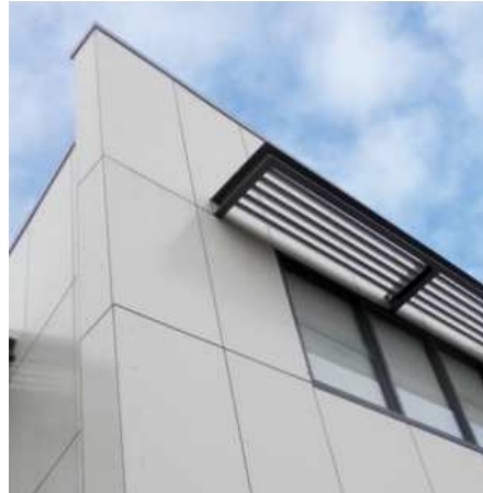
CFC01 - COMPRESSED FIBRE CEMENT
