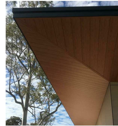
CLG13 - ALUMINIUM SOFFIT LINING
