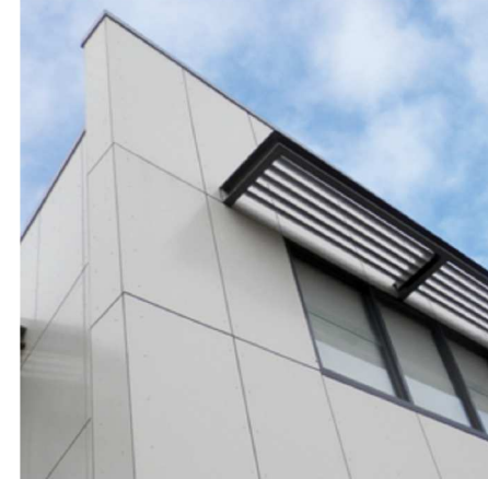
CFC01 - COMPRESSED FIBRE CEMENT
