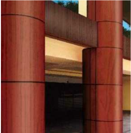
MC01 - ALUMINIUM CLADDING AROUND STEEL COLUMNS
