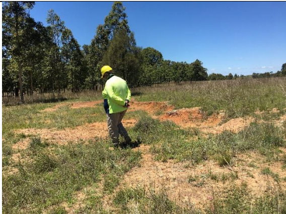
Photo 11 – erosion scald adjacent LID34
