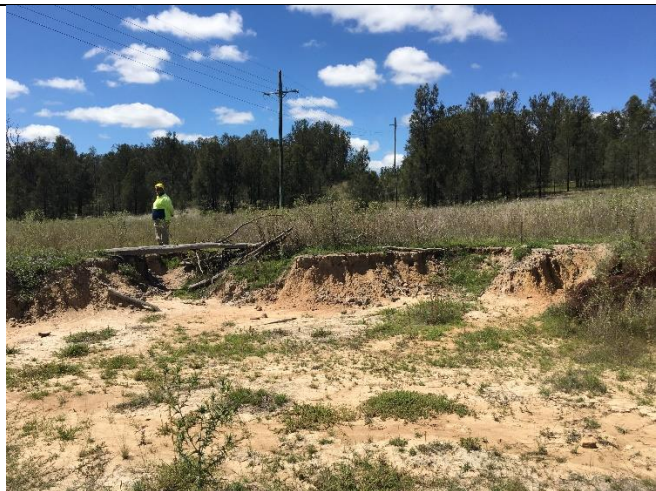
Photo 6 – LID3 erosion & old fencing materials in gully
