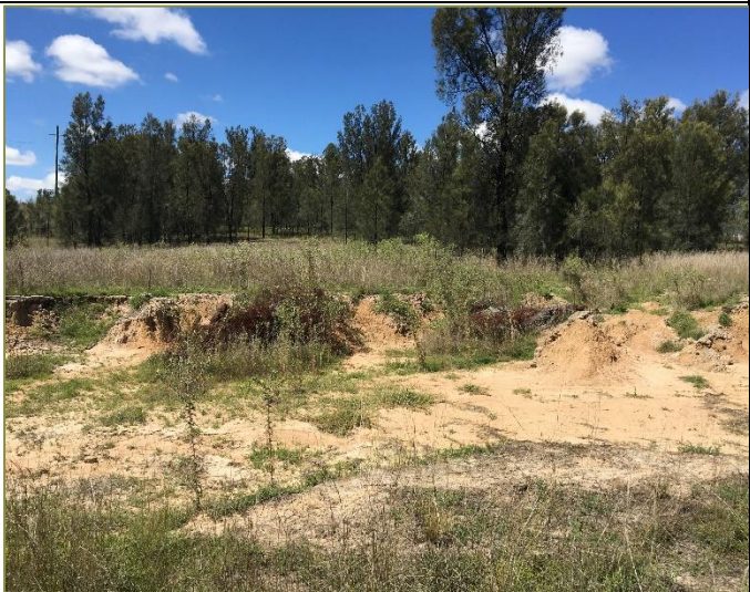
Photo 4 – LID3 erosion monitoring
