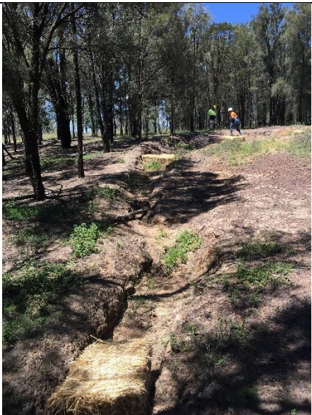
Photo 9 – erosion gully at HAZ2-OS1
