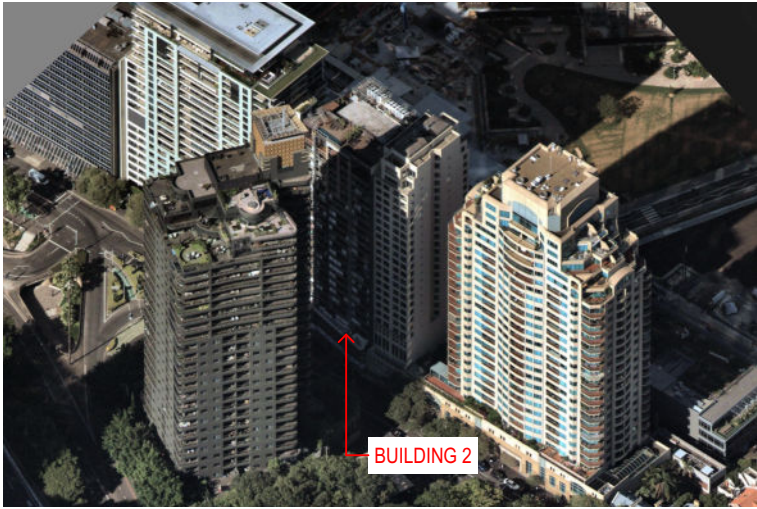
○ AERIAL VIEW Building 2
