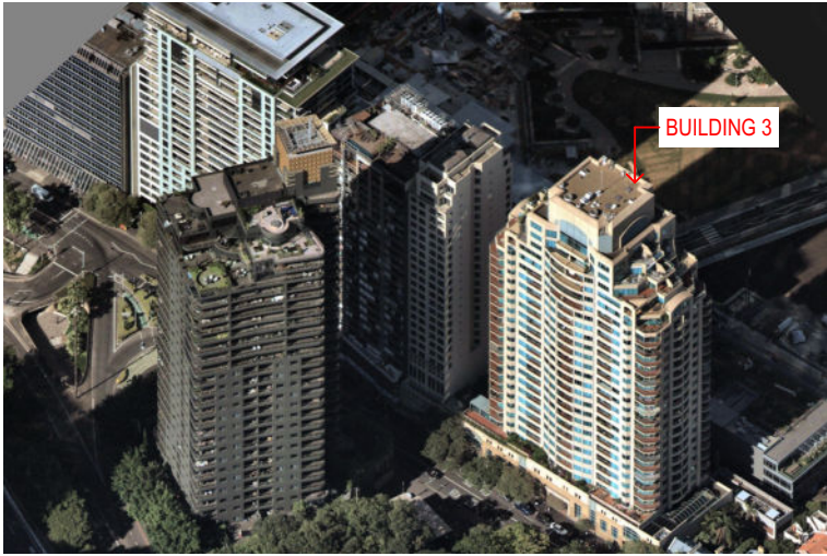
AERIAL VIEW Building 3
