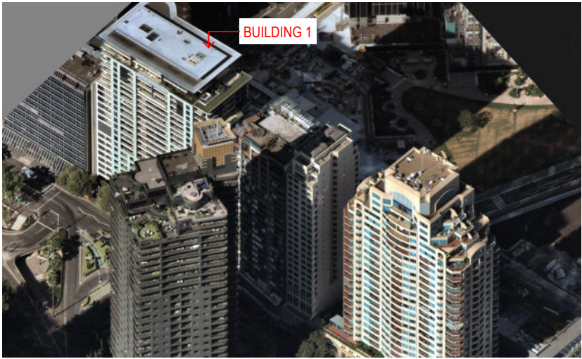
○ AERIAL VIEW Building 1
