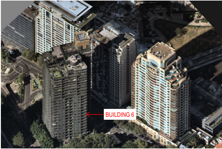
AERIAL VIEW Building 6
