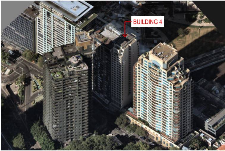
AERIAL VIEW Building 4
