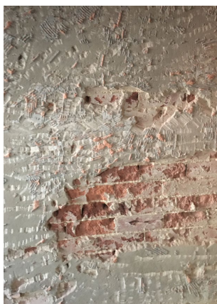
Figure 6 – Previously obscured later brick wall to basement level.
