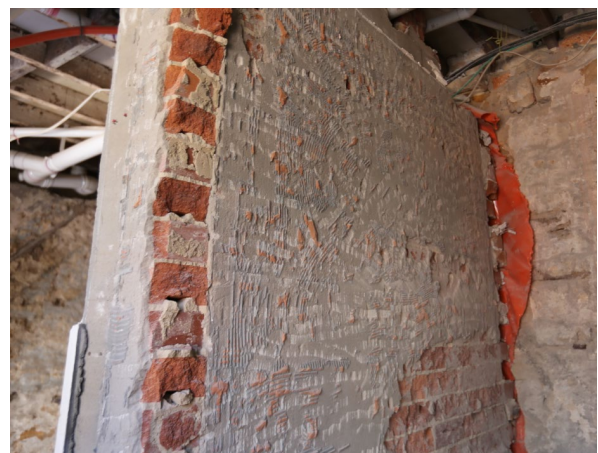
Figure 7 – Previously obscured later brick wall to basement level.
