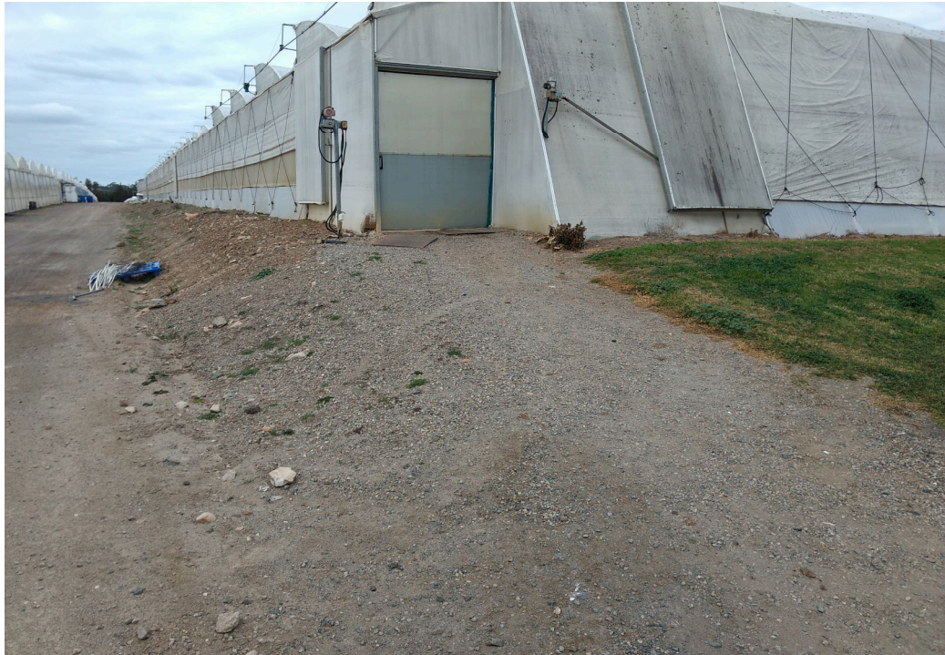
Photograph 7 - Typical fill placed for greenhouse construction
