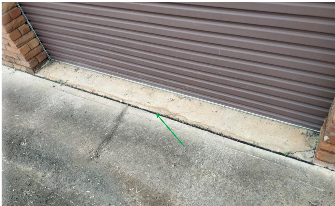
Photograph 11. 31B main building external, bituminous membrane between concrete joints, no asbestos detected, as observed on 18/01/2022.
