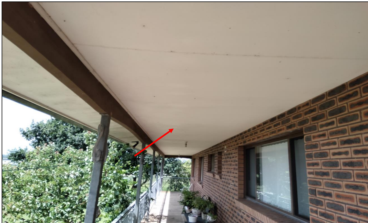
Photograph 6. Building external, all around, eaves and awnings, chrysotile asbestos containing fibre cement sheeting, as observed on 18/01/2022.
