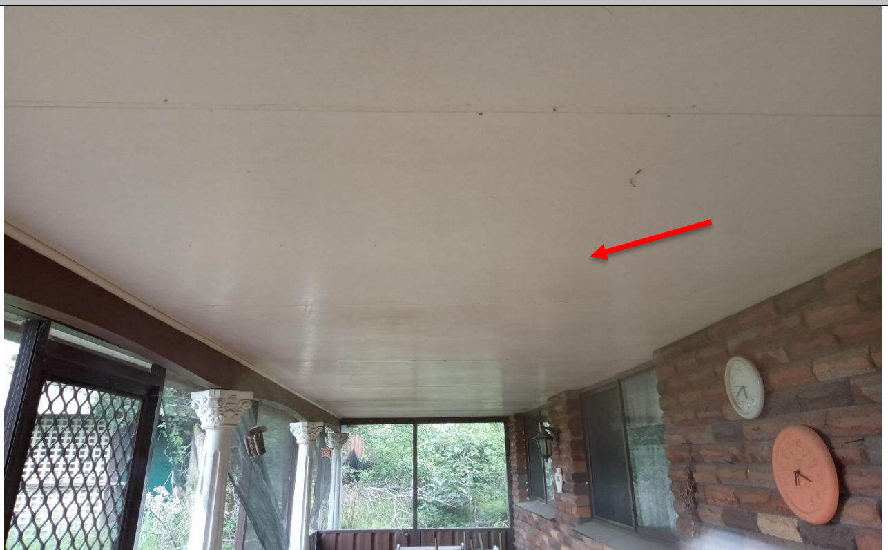
Photograph 4. Internal, front and rear entrance - asbestos containing ceiling lining, as observed on 12/01/2022.
