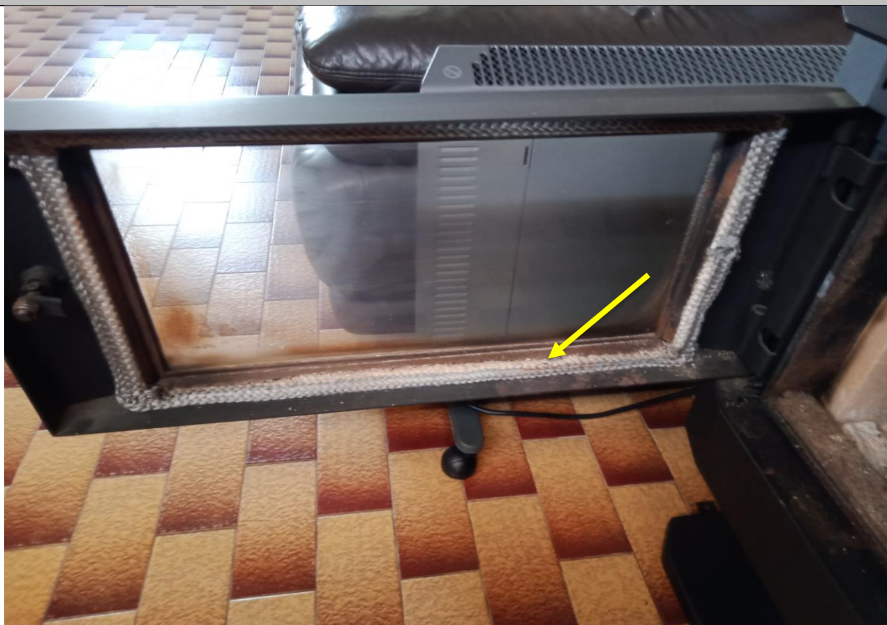
Photograph 2. West building, Internal, ground, living room, non-asbestos containing, SMF fibres detected rope seal to furnace door, as observed on 12/01/2022.
