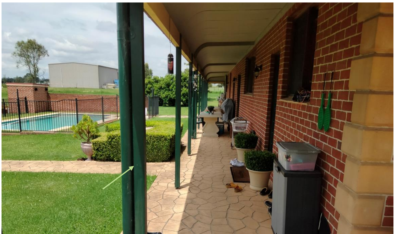
Photograph 4. 31A Main building, northern and eastern side, beams supporting eaves and awnings, non-lead containing green paint system, as observed on 18/01/2022.
