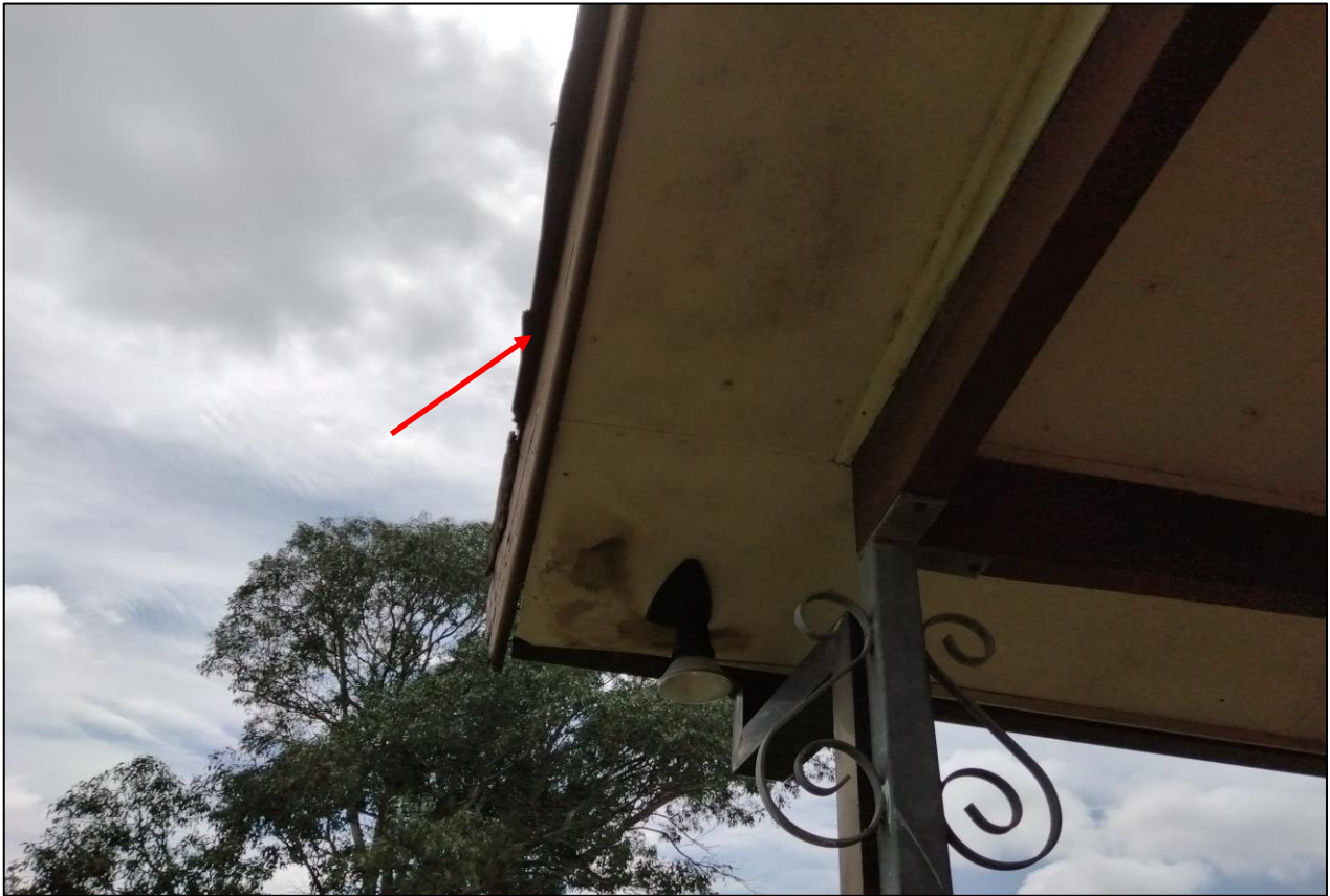
Photograph 7. Building external, panel beneath roof, Chrysotile asbestos containing fibre cement panel, as observed on 18/01/2022.
