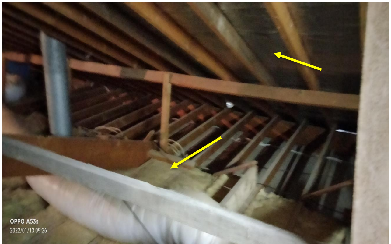
Photograph 5. Internal, main building, ceiling void – presumed SMF sarking and insulation batts as observed on 12/01/2022.
