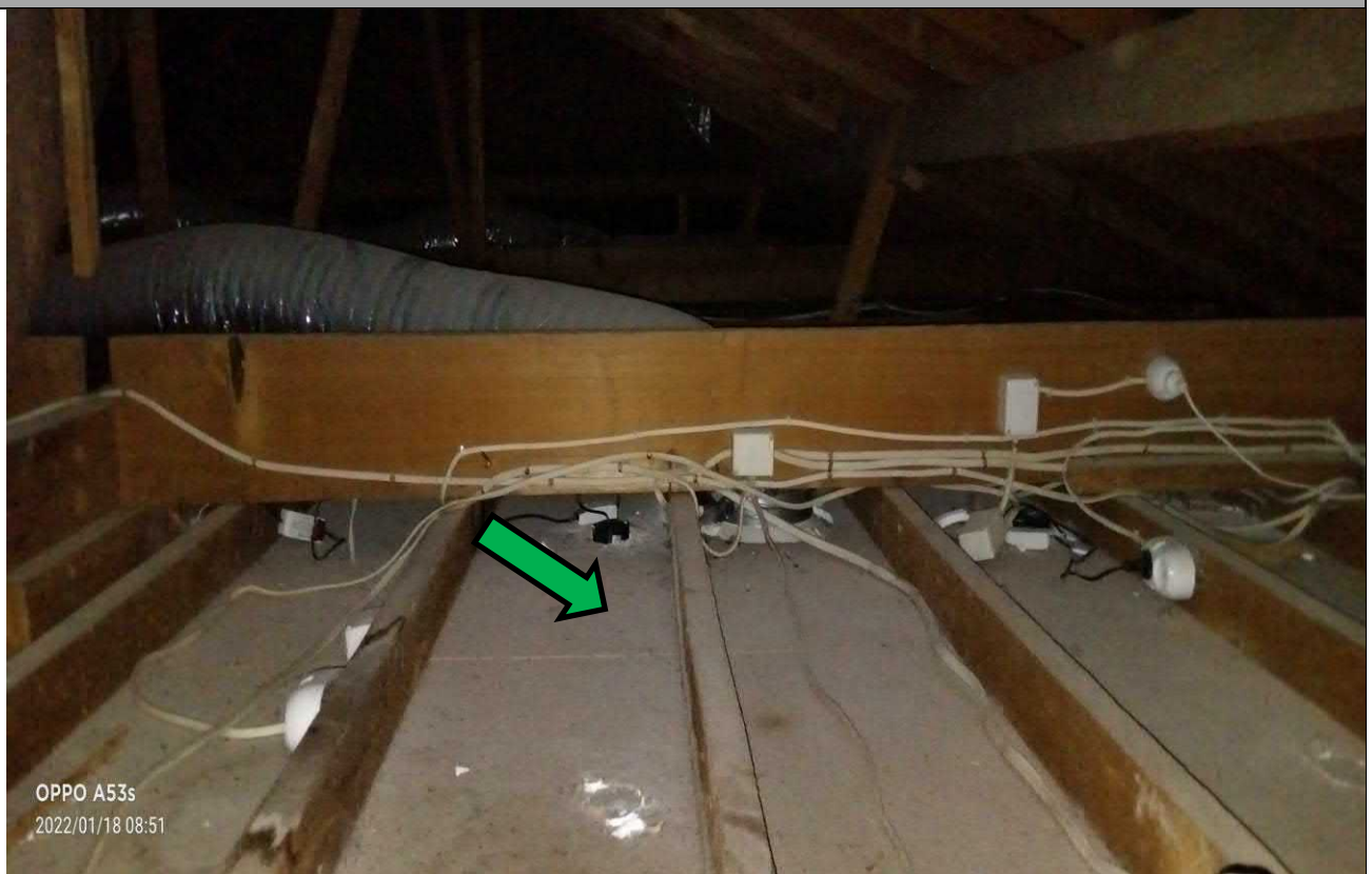
Photo 2: Main building, ceiling space, non-asbestos containing dust, as observed on 18/01.2022.
