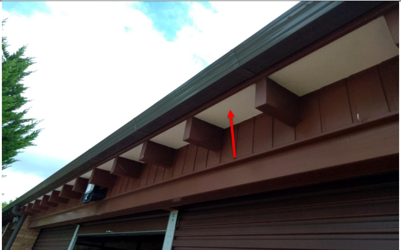
Photograph 5. West building, external, asbestos containing FC eaves lining, as observed on 12/01/2022.
