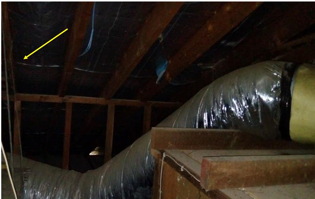
Photograph 9. 31B main building Internal, ceiling void – presumed SMF sarking, as observed 18/01/2022.
