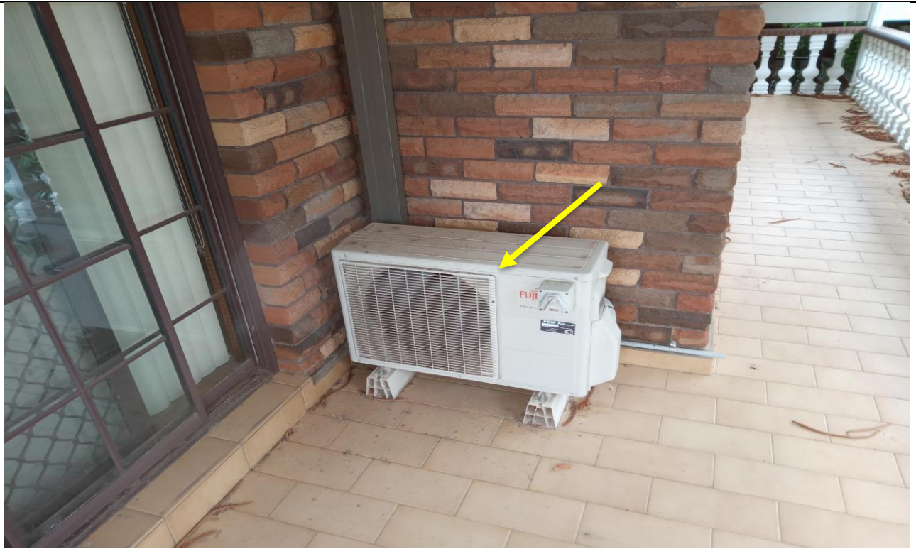
Photograph 7. External front balcony, non ODS gas R32, as observed on 12/01/2022.
