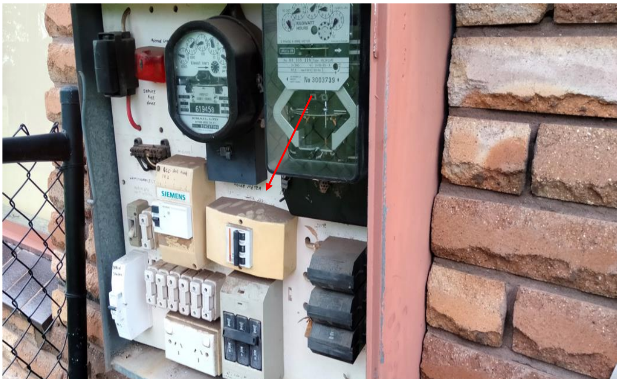
Photograph 14. 31B main building external, north western side, electrical backing panel, presumed to contain asbestos, as observed on 18/01/2022.
