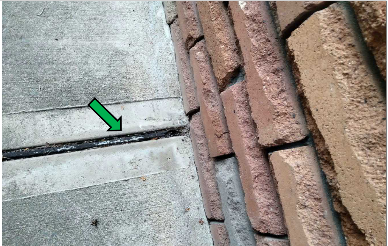
Photo 5: Modern building, expansion joints, non-asbestos containing mastic, as observed on 18/01/2022.
