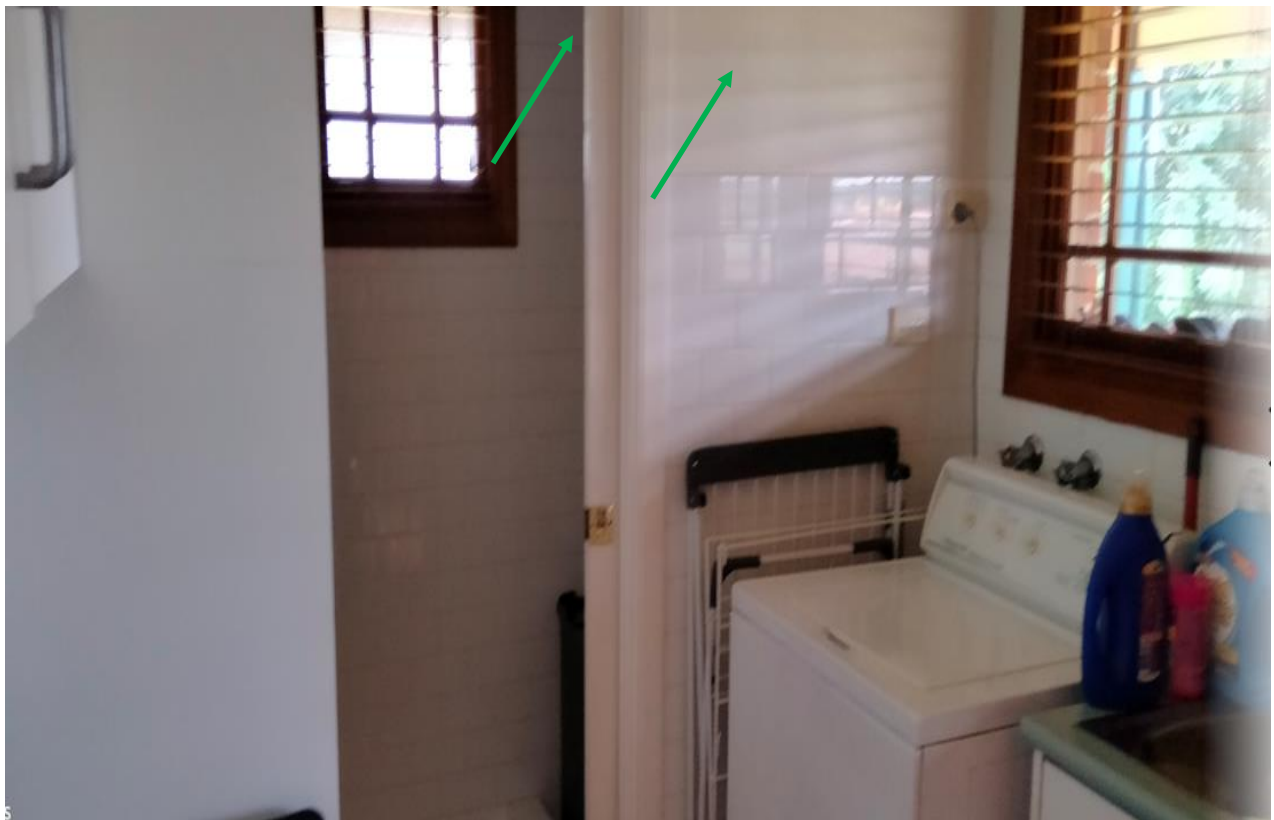
Photograph 3. 31A Main building internal, northeaster bathroom, walls, non-asbestos fibre cement sheeting, as observed on 18/01/2022.
