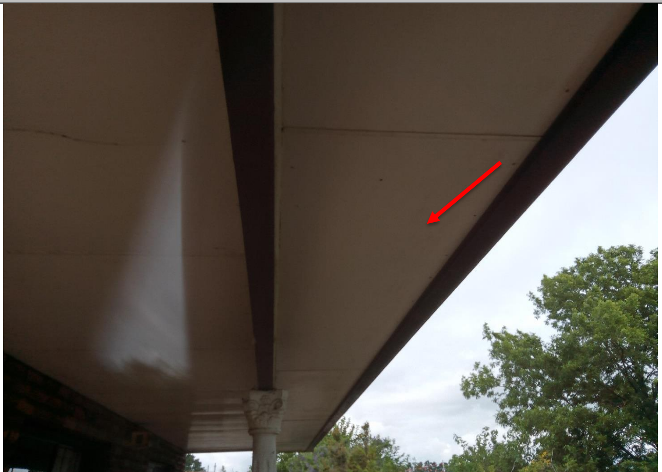
Photograph 2. External eaves, asbestos containing fibre cement, as observed on 12/01/2022.
