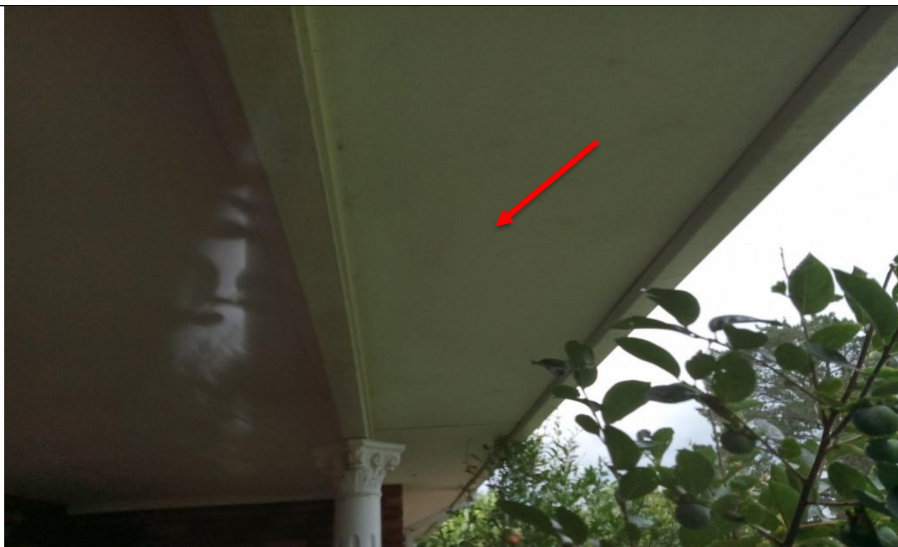
Photograph 1. 198B residence, External surround, asbestos containing eaves lining, as observed on 12/01/2022.
