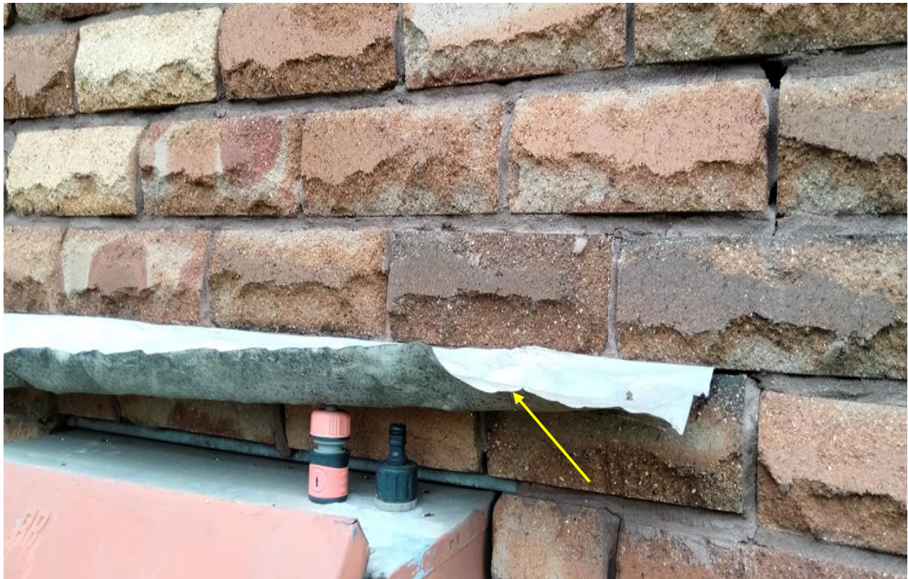
Photograph 15. 31B main building external, north western side, above electrical backing panel, lead flashing, as observed on 18/01/2022.
