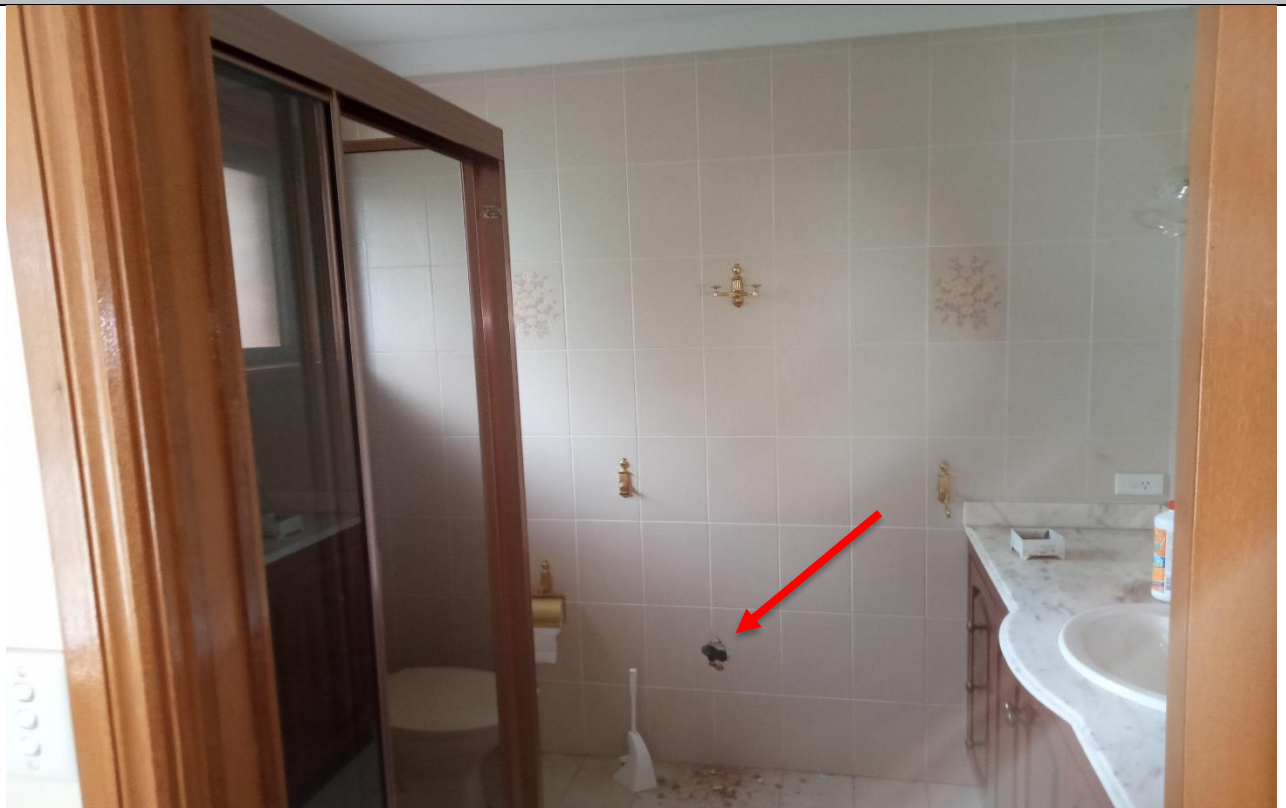
Photograph 6. Internal, bathroom ensuite wall lining, sbestos containing fibre cement, as observed on 12/01/2022.
