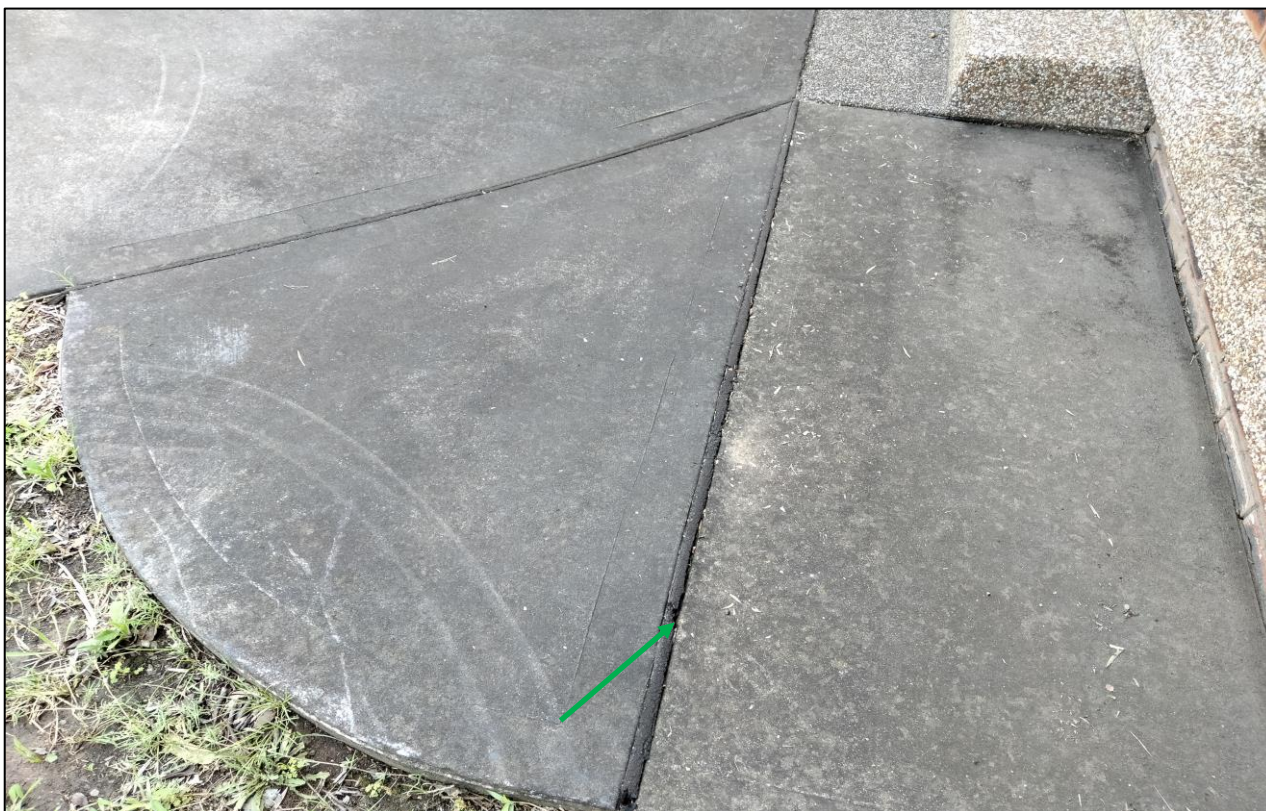
Photograph 2. Building external, bituminous material between concrete joints, no asbestos detected, as observed on 18/01/2022.
