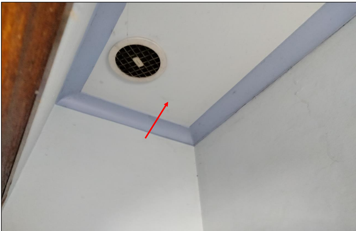
Photograph 3. Building internal, toilet and bathroom, ceiling, chrysotile asbestos containing fibre cement sheeting, as observed on 18/01/2022.
