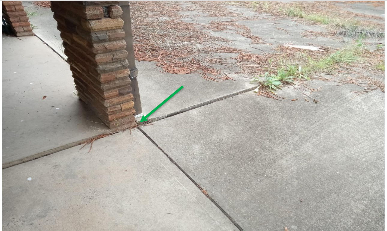
Photograph 1. External surround, non asbestos Bitumen mastic to concrete slab, as observed on 12/01/2022.
