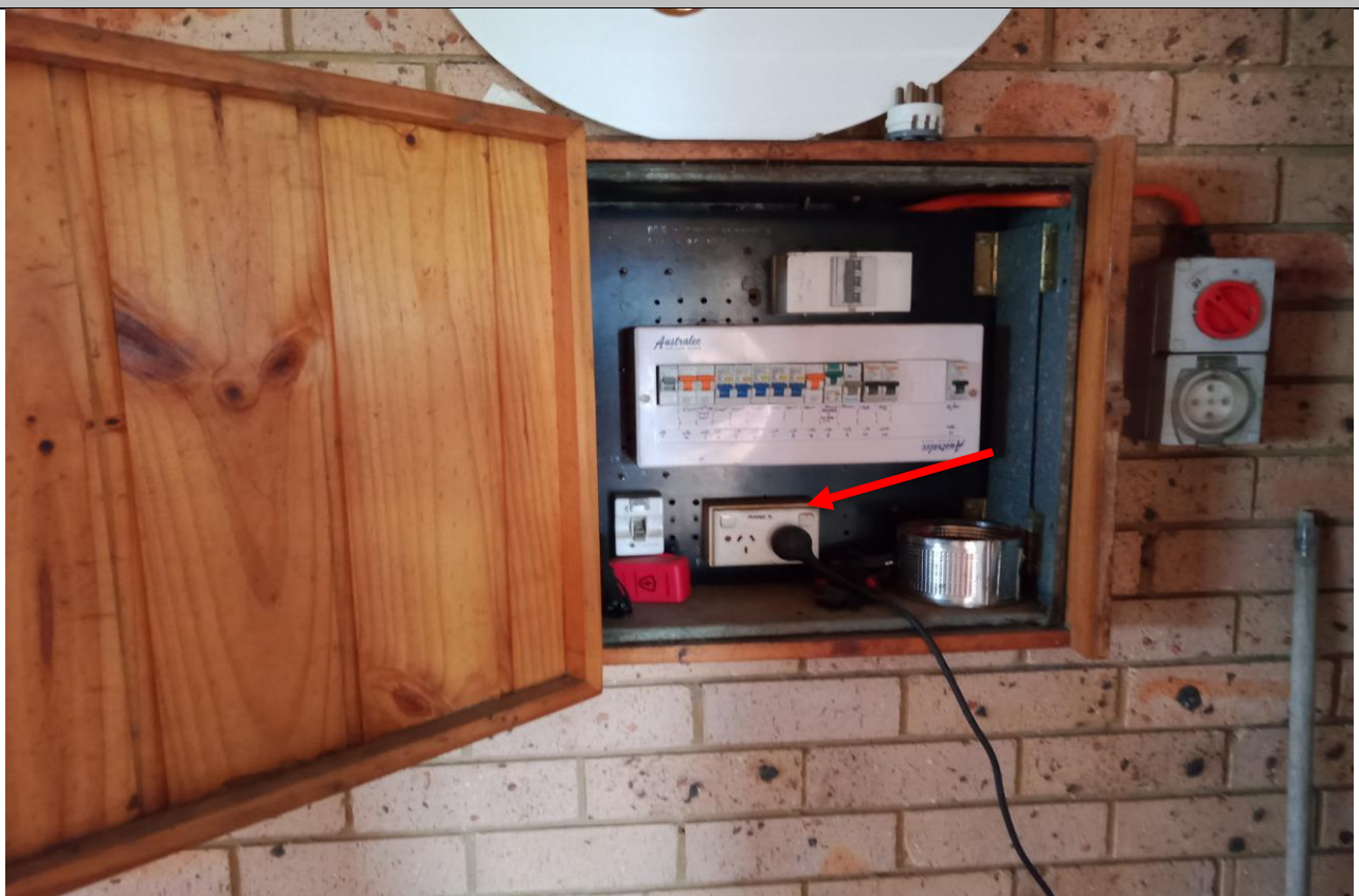
Photograph 4. West building, Internal, ground, presumed asbestos containing electrical backing board, as observed on 12/01/2022.
