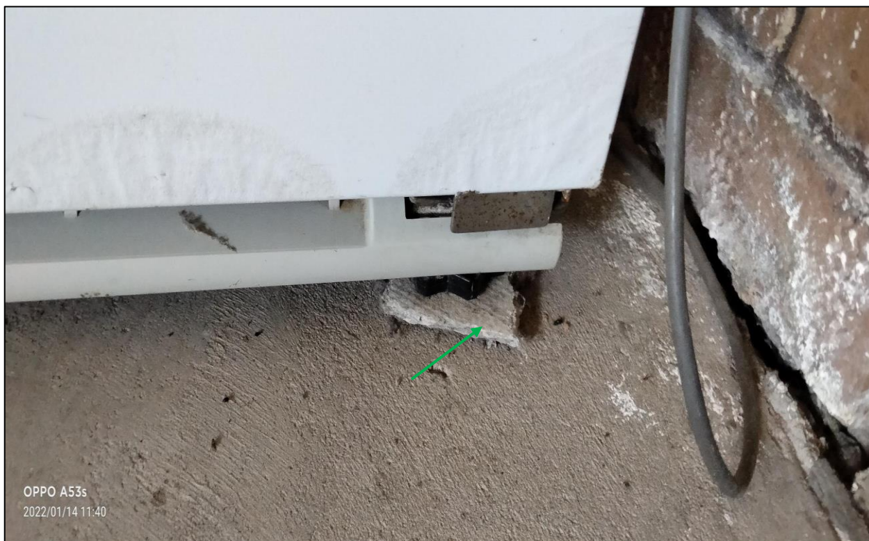
Photograph 5. Building internal, garage, non-asbestos containing independent fibre cement fragment used as part, as observed on 18/01/2022.
