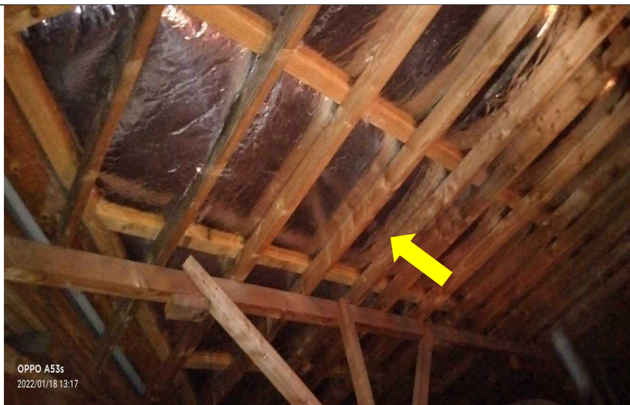
Photo 5: Main building, ceiling, sarking insulation, presumed SMF, as observed on 18/01/2022.
