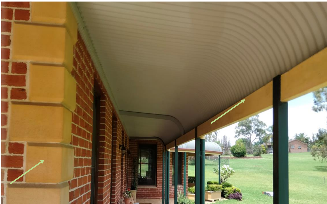
Photograph 5. 31A Main building, northern and eastern side, beams to gutter lining and walls, non-lead containing cream paint system, as observed on 18/01/2022.
