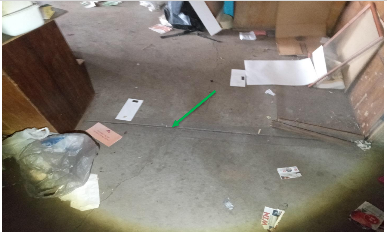
Photograph 5. Internal, ground level, non asbestos bitumen mastic to concrete floor slabs, as observed on 12/01/2022.
