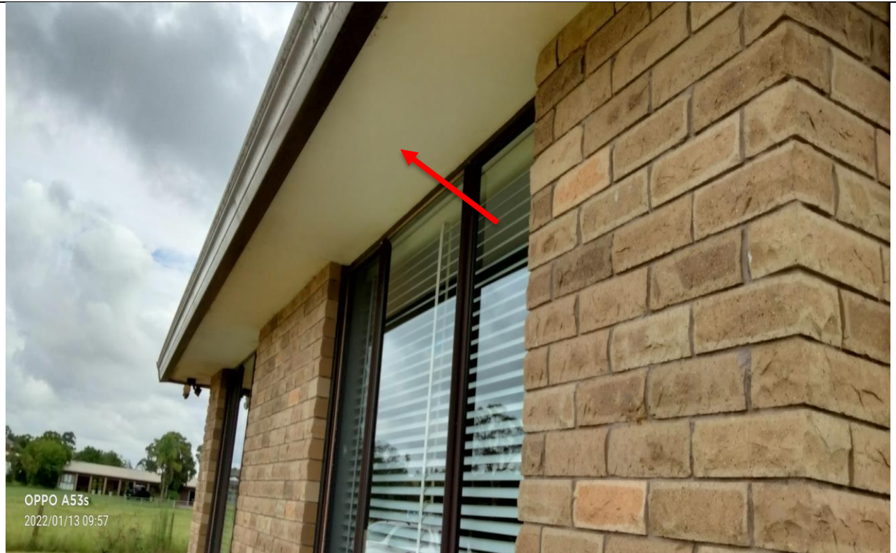
Photograph 3. 198A residence, External surround, asbestos containing eaves lining, as observed on 12/01/2022.
