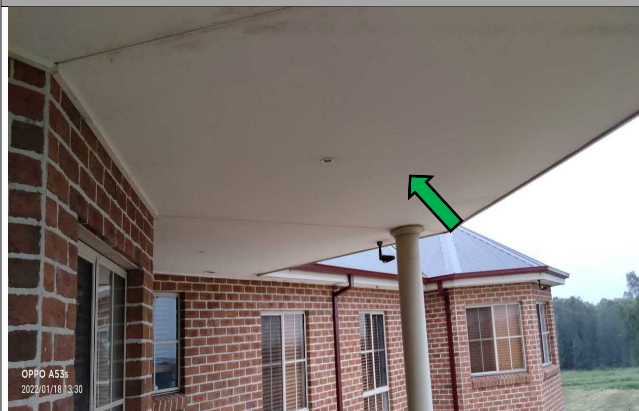
Photo 2: Main building, eaves, non-asbestos containing fibre cement sheeting, as observed on 18/01/2022.
