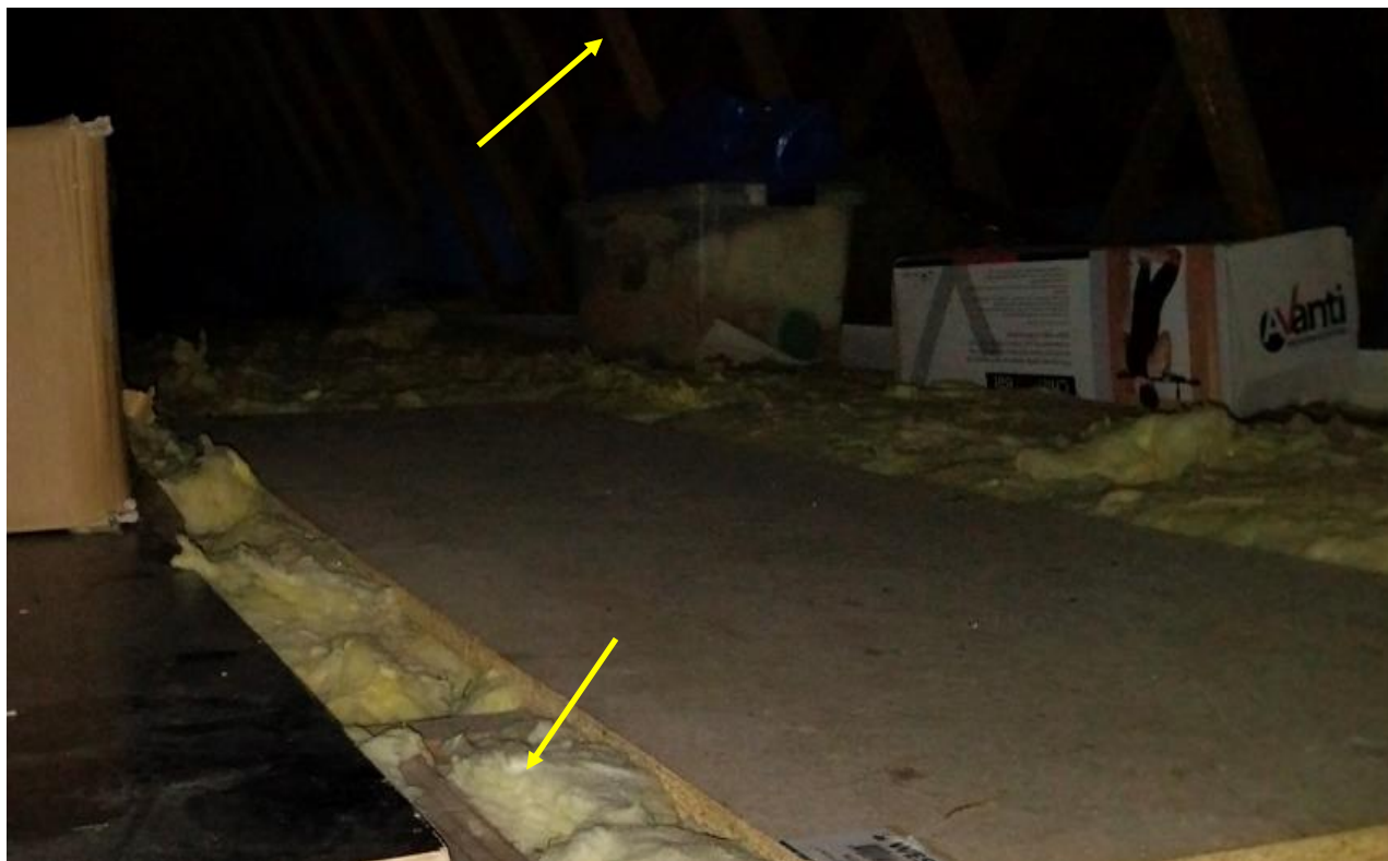
Photograph 2. 31A Main building internal, ceiling space, insulation, no asbestos detected, SMF detected, as observed on 18/01/2022.
