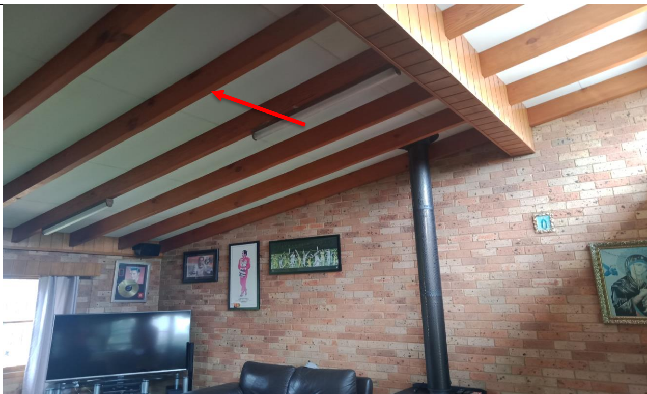
Photograph 1. West building, Internal, ground, living room, asbestos containing FC ceiling lining, as observed on 12/01/2022.
