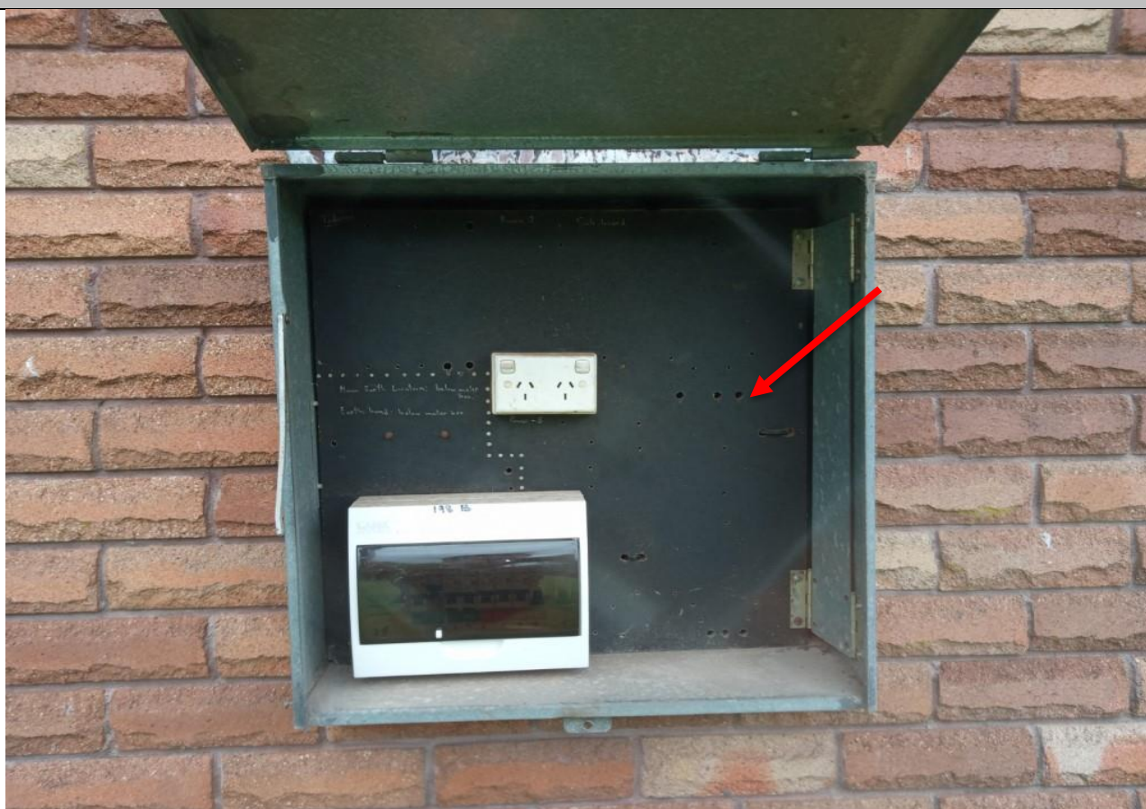
Photograph 2. 198B residence, External, presumed asbestos containing electrical backing board, as observed on 12/01/2022.
