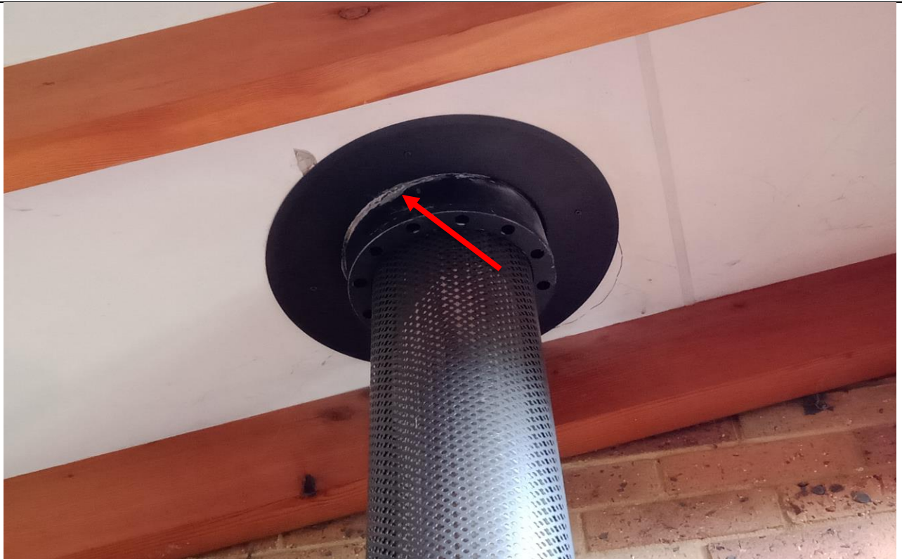
Photograph 3. West building, Internal, ground, living room, asbestos containing mastic to furnace flue pipe, as observed on 12/01/2022.
