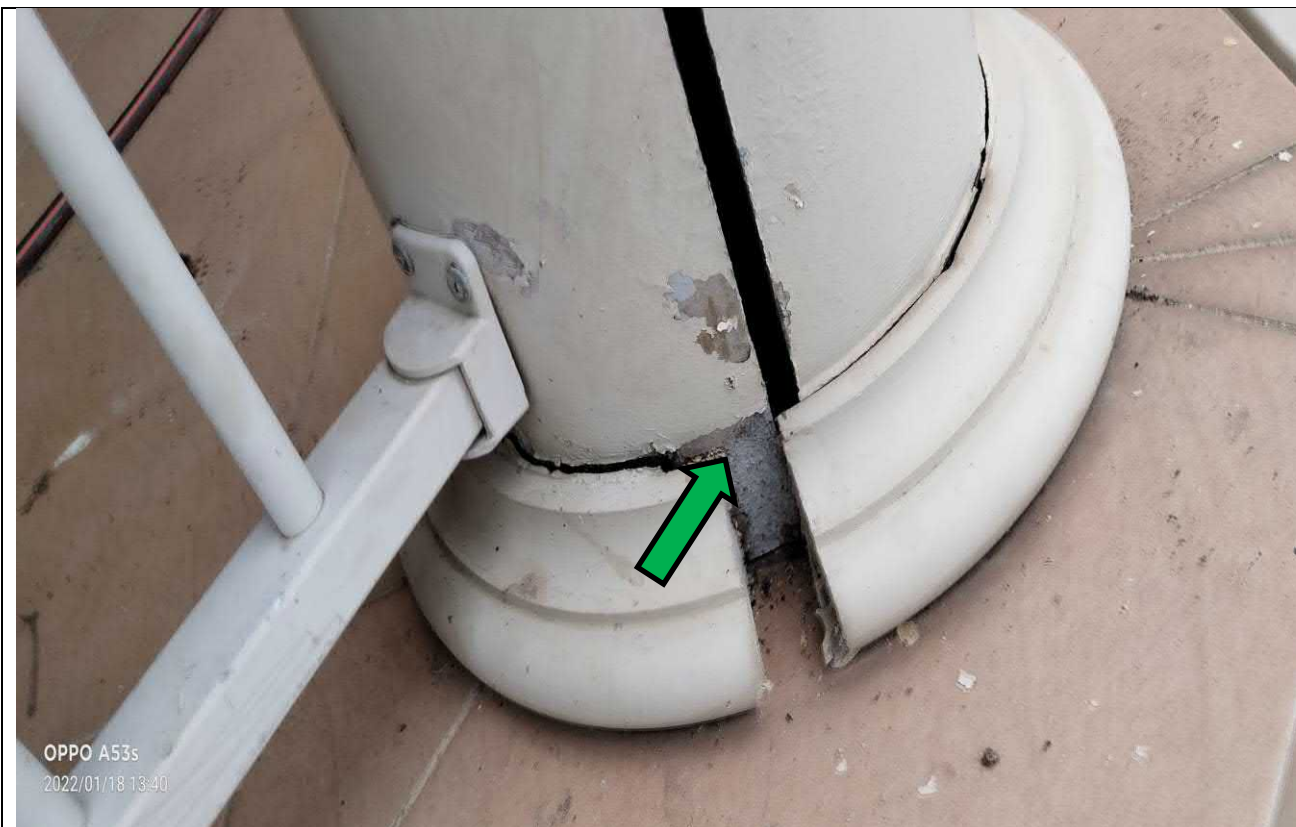
Photo 3: Main building, pillars, non-asbestos containing moulded fibre cement sheeting, as observed on 18/01/2022.
