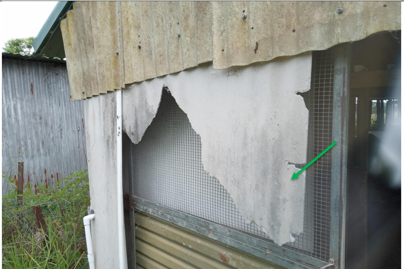
Photograph 3. External, storage and animal cages wall lining and entrance door, non-asbestos containing fibre cement, as observed on 12/01/2022.
