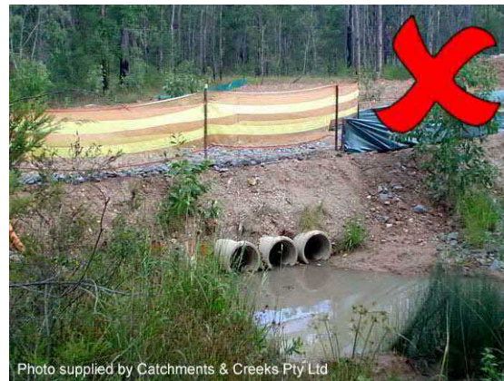
Photo 4 – If the culvert has insufficient hydraulic capacity, then overtopping flows are likely to cause severe bank erosion
