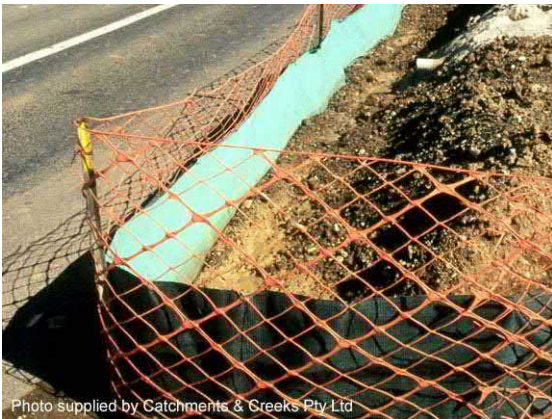
Photo 25 – Installation with safety fencing used as support
