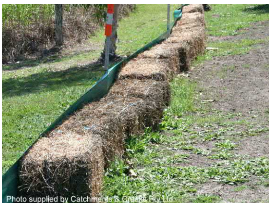
Photo 17 – Straw bales placed up-slope of fence to separate sediment and fabric
