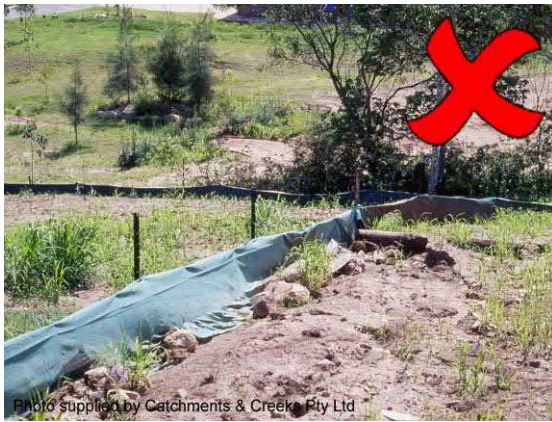
Photo 29 – Flow diversion by fence
