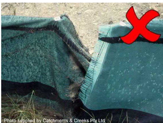
Photo 19 – Inappropriate junction
