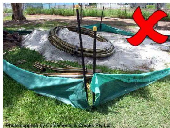
Photo 20 – Gaps in fence are not allowed
