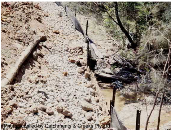
Photo 39 – Spill-through weir with up-slope aggregate filter
