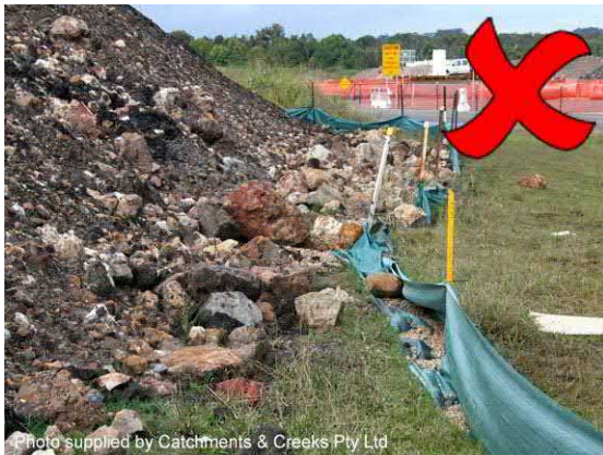
Photo 31 – Damage by shifting fill
