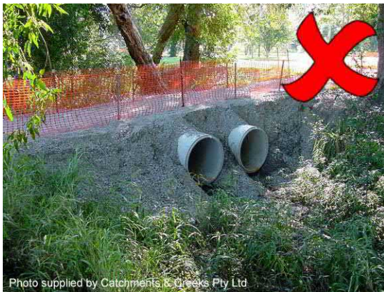
Photo 3 – Using only fine aggregate to form the fill embankment can result in severe wash-outs if overtopped
