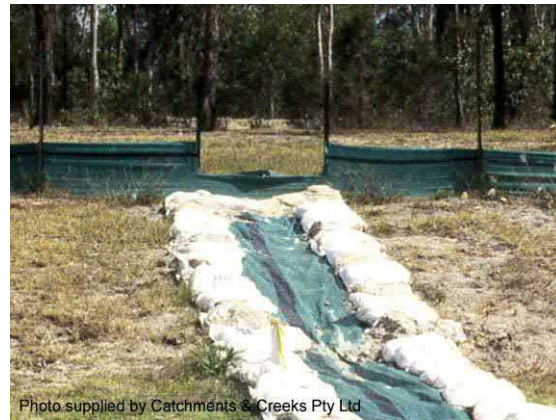
Photo 38 – Spill-through weir with outlet chute
