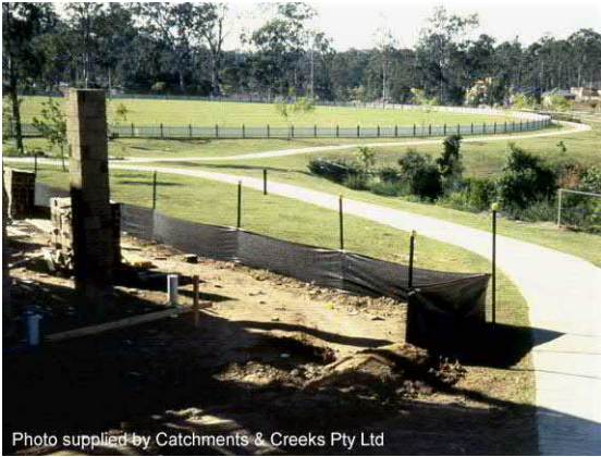
Photo 21 – Installation without backing weir/mesh
