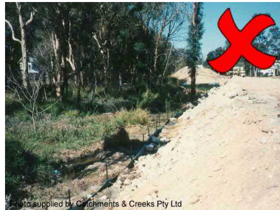
Photo 32 – Fence placed too close to fill
