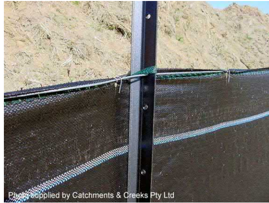
Photo 22 – Installation with top wire support
