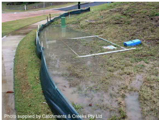
Photo 9 – Sediment fence placed along the contour
