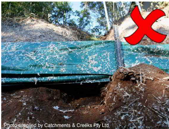
Photo 33 – Evidence of hydraulic wash-out under fence caused by poor trenching
