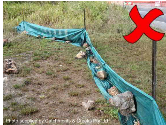
Photo 14 – Inappropriate installation
