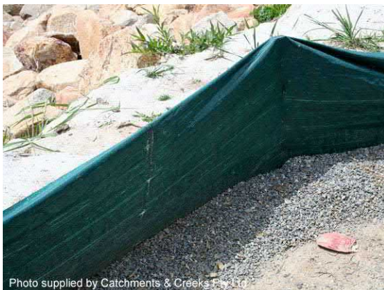
Photo 15 – Bottom of fabric buried under aggregate
