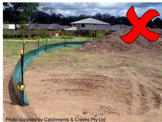
Photo 18 – Inappropriate installation of the posts up-slope of the fabric
