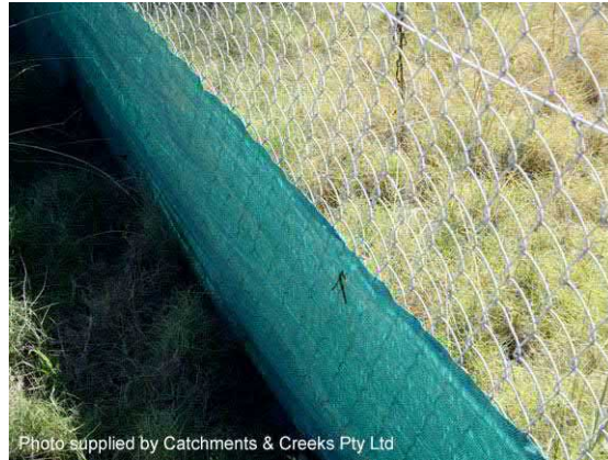
Photo 24 – Installation using fence support
