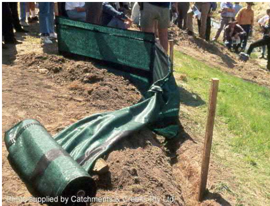
Photo 13 – Trenching the fabric
