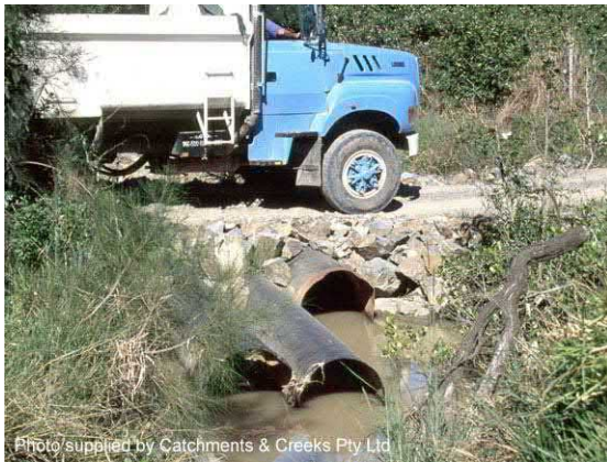
Photo 1 – Temporary culvert formed from recycled steel pipes
