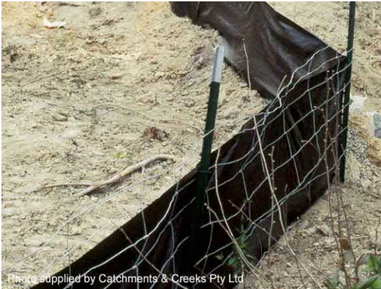
Photo 23 – Installation with weir mesh
