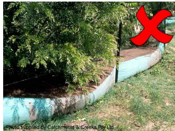
Photo 34 – Sediment not removed after storm
