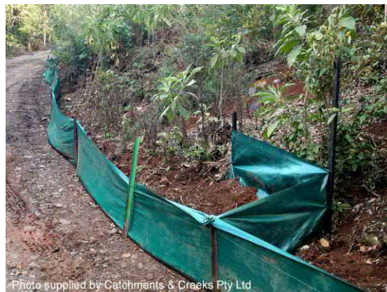
Photo 12 – Alternative design of a fence 'return'
