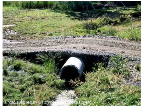
Photo 2 – Temporary crossing of minor drainage channel
