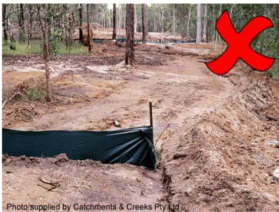
Photo 35 – Flow allowed to bypass the fence
