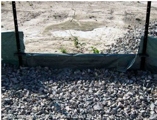
Photo 37 – Spill-through weir (down-slope side) with rock splash pad
