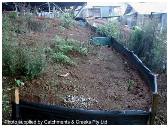
Photo 11 – Placement of fence off the contour with regular fence 'returns'
