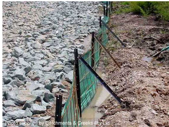
Photo 26 – A sediment fence braced for possible high flows
