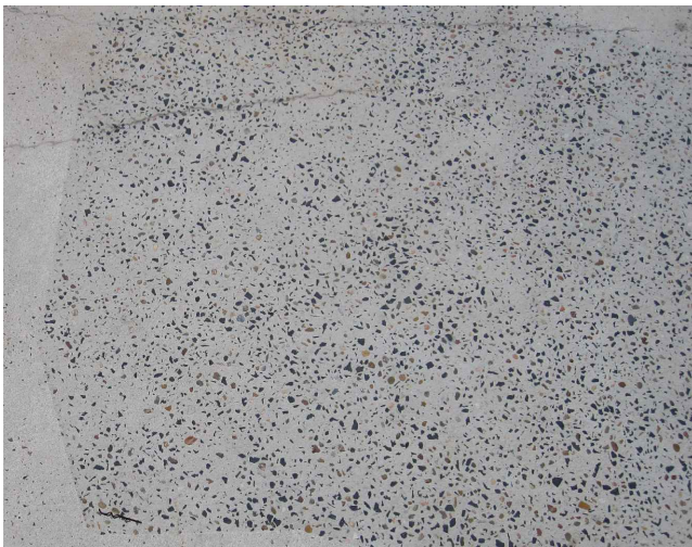
PV01: INSITU CONCRETE PAVING, EXPOSED AGGREGATE
