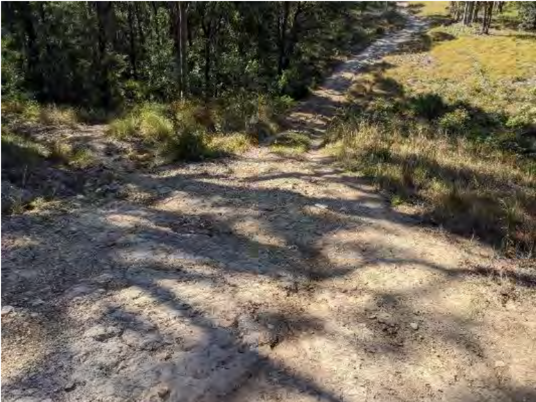
Plate 6.9 Example of erosion and topsoil disturbance as a result of ongoing track use on the slope in SU4
