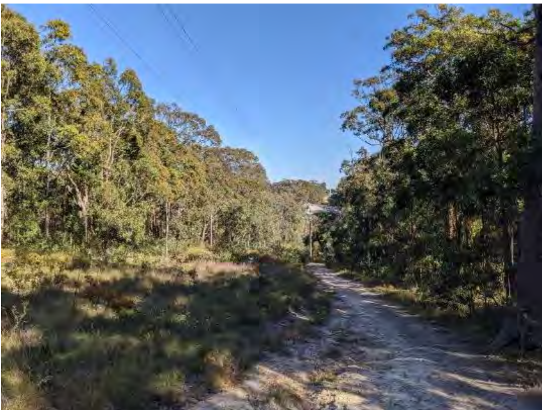
Plate 6.10 Example of site disturbance as seen through the eroded dirt track, vegetation clearance and overhead powerline within a powerline easement in SU4
