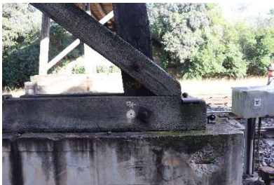
Bridge on Mathews Lane
