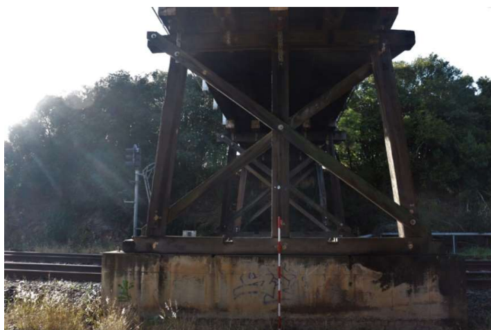
East facing view of underside of Bridge on Mathews Lane showing timber cross bracing and concrete foundations.
