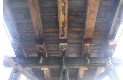
Bridge on Mathews Lane
