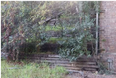
Prince Street Overbridge
