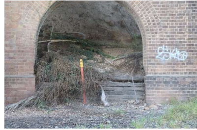
Prince Street Overbridge
