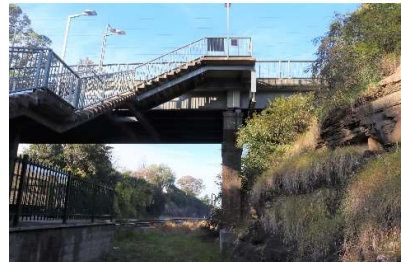
Prince Street Overbridge
