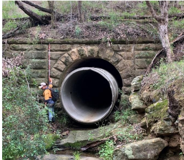
Plate 3.6 Sandstone culvert 88.980 with RCP sleeve.
