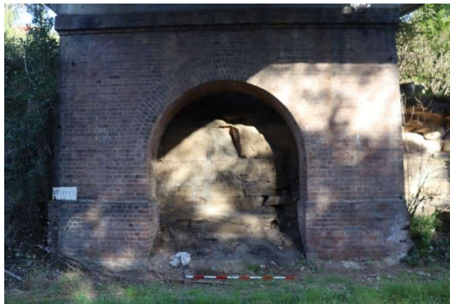
WSW facing view of Prince Street Overbridge showing brick arched piers and railway cutting (into sandstone bedrock).
