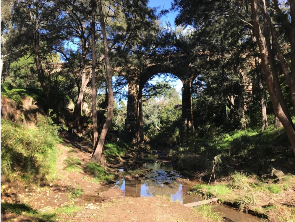
Plate D.10 Looking south-west towards Picton Viaduct from Stonequarry Creek.
