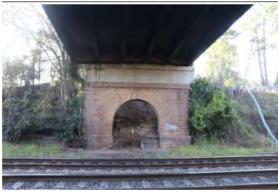
Prince Street Overbridge
