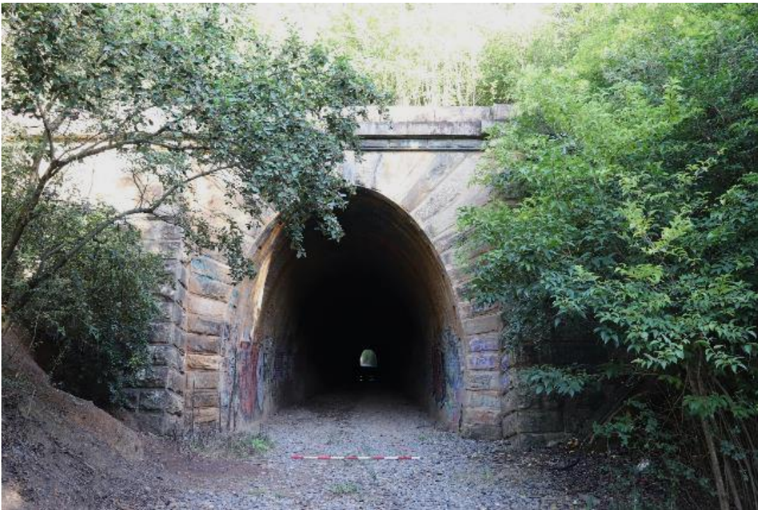
Plate D.6 Mushroom Tunnel, southern entrance. Dressed sandstone blocks radiate from the portal. View north-west.
