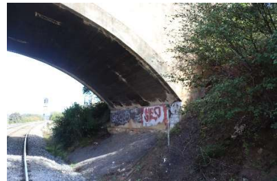
Connellan Crescent Overbridge
