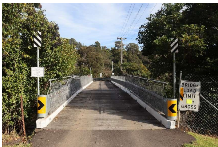
East facing view of Bridge on Mathews Lane showing timber decking, metal guard rails and modern signage.
