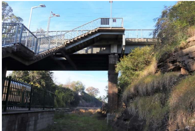
Southeast facing view of the Prince Street Overbridge from within the Main Southern Railway corridor showing brick piers and pedestrian access staircase.
