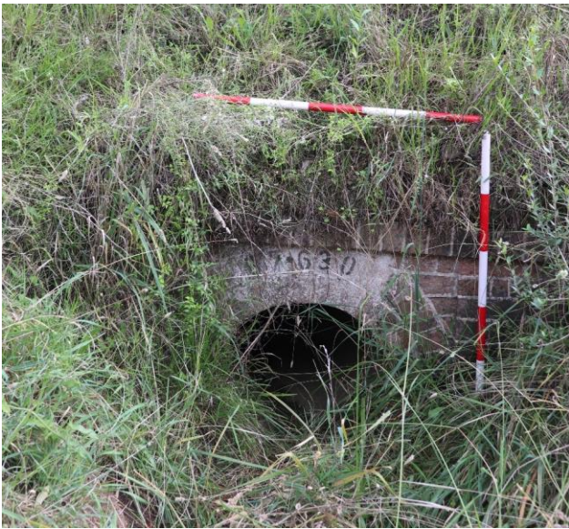
Plate 3.3 Brick culvert (chainage 87.630). View north-west.
