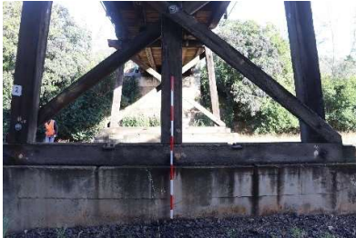
Bridge on Mathews Lane
