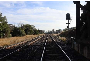
Bridge on Mathews Lane
