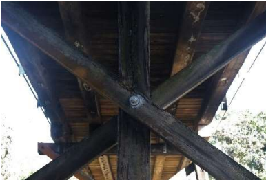
Bridge on Mathews Lane
