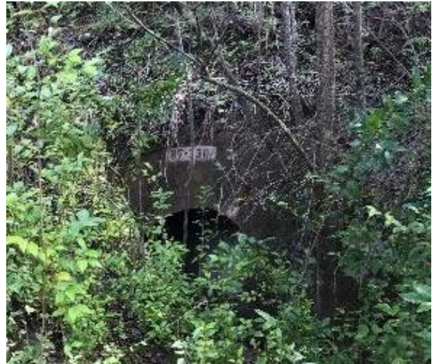
Plate 3.2 Culvert 87.330 km. View north-west.
