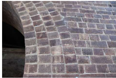
Prince Street Overbridge
