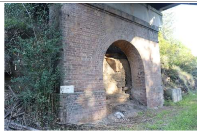
Prince Street Overbridge
