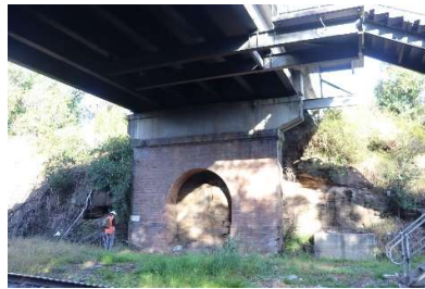
Prince Street Overbridge
