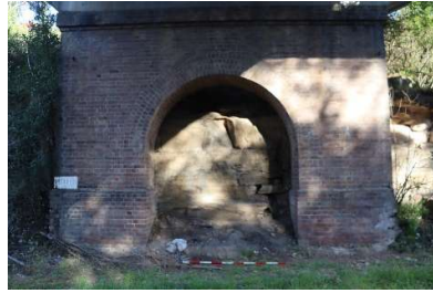
Prince Street Overbridge
