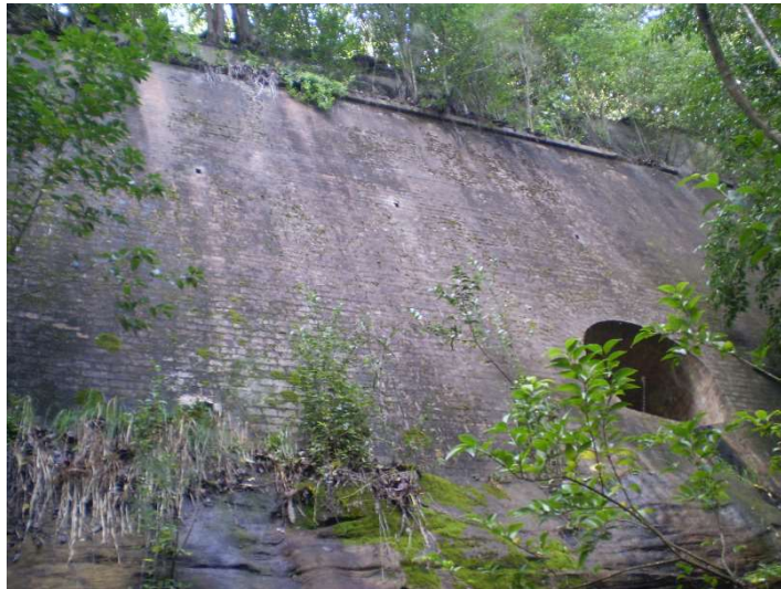
East facing view of high retaining wall from Stonequarry Creek.
