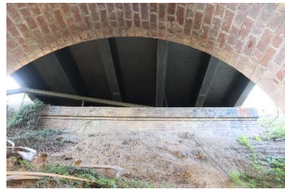
Prince Street Overbridge
