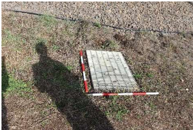
Concrete drain at chainage 87.918km
