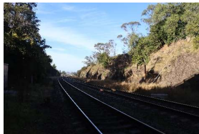
Prince Street Overbridge
