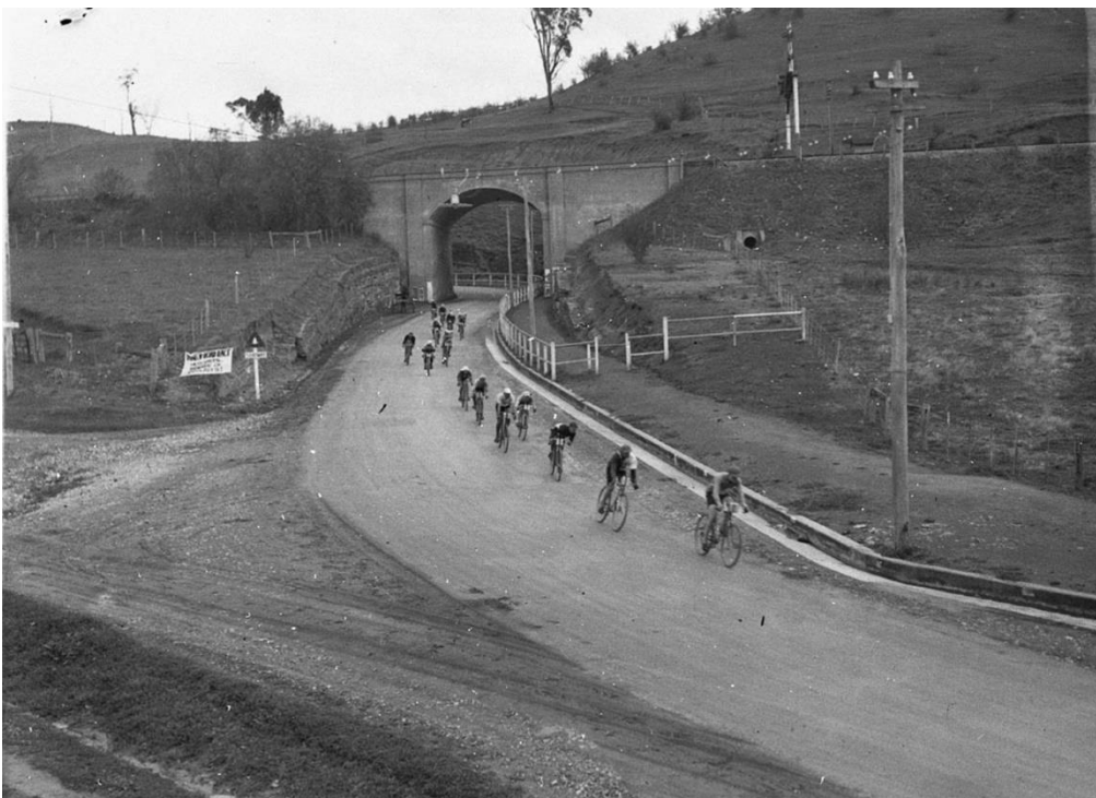
Plate D.13 ‘A line of cyclists coming through the arch of the railway bridge at Picton’, Sam Hood, 1930 (SLNSW Home and Away 2473). View west.
