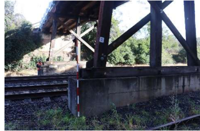
Bridge on Mathews Lane
