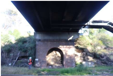
Prince Street Overbridge
