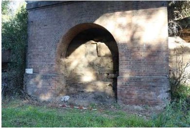
Prince Street Overbridge
