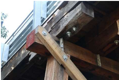
Bridge on Mathews Lane
