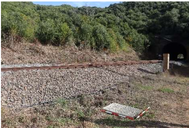
Concrete drain at chainage 87.918km
