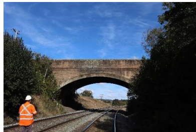
Connellan Crescent Overbridge
