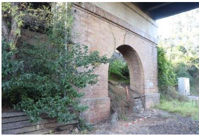
Prince Street Overbridge
