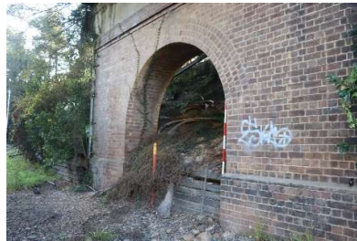
Prince Street Overbridge
