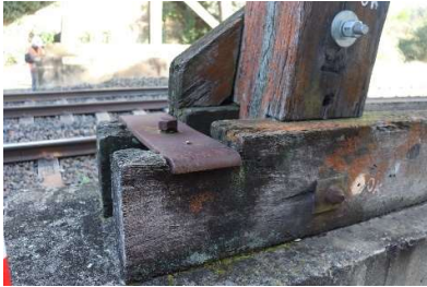
Bridge on Mathews Lane
