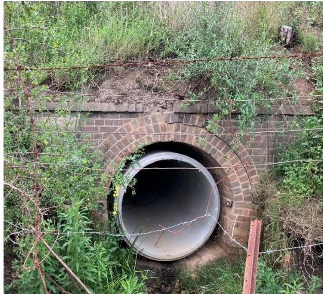
Plate 3.4 Brick culvert (chainage 87.850). View north-west.
