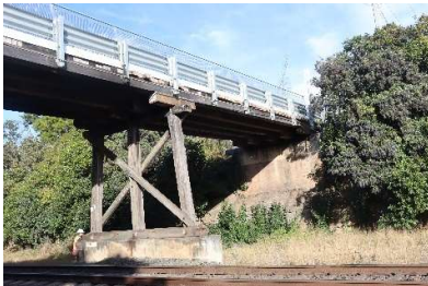
Bridge on Mathews Lane
