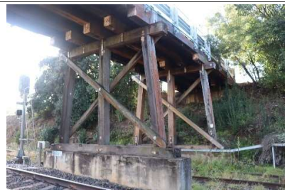
Bridge on Mathews Lane
