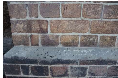
Prince Street Overbridge
