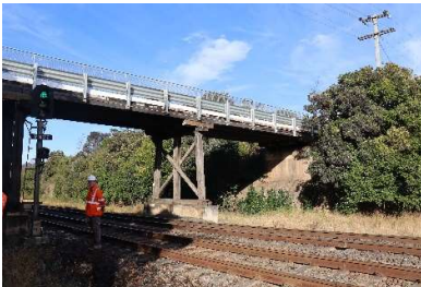
Bridge on Mathews Lane
