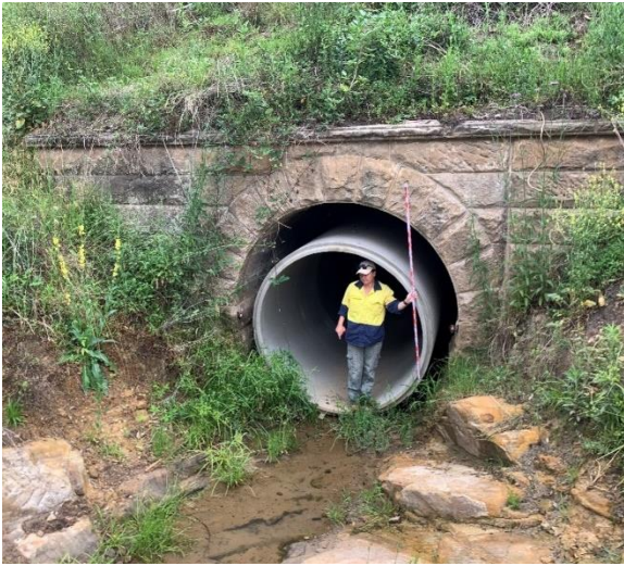
Plate 3.5 Sandstone culvert 88.400 with RCP sleeve (The RCP is a mitigation measure for subsidence, refer to Table 6.1).
