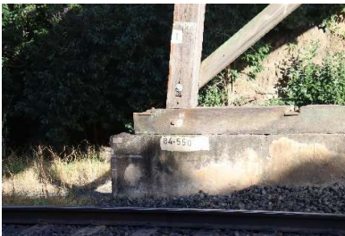
Bridge on Mathews Lane
