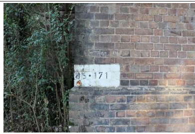
Prince Street Overbridge
