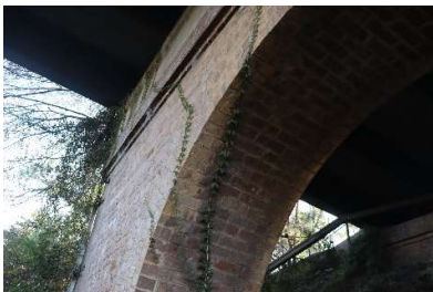
Prince Street Overbridge
