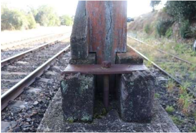
Bridge on Mathews Lane
