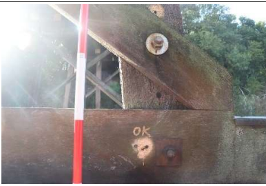
Bridge on Mathews Lane
