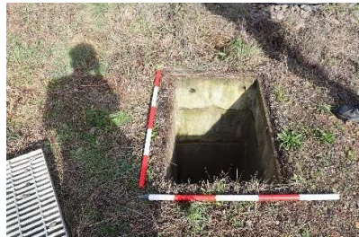
Concrete drain at chainage 87.918km
