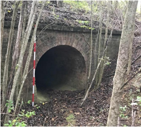
Plate 3.1 Brick culvert (chainage 87.300) beneath disused embankment. View east.
