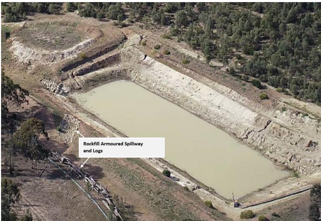
Plate 2: NOOP1 Sediment Dam Spillway Outfall with Level Spreader and Logs
