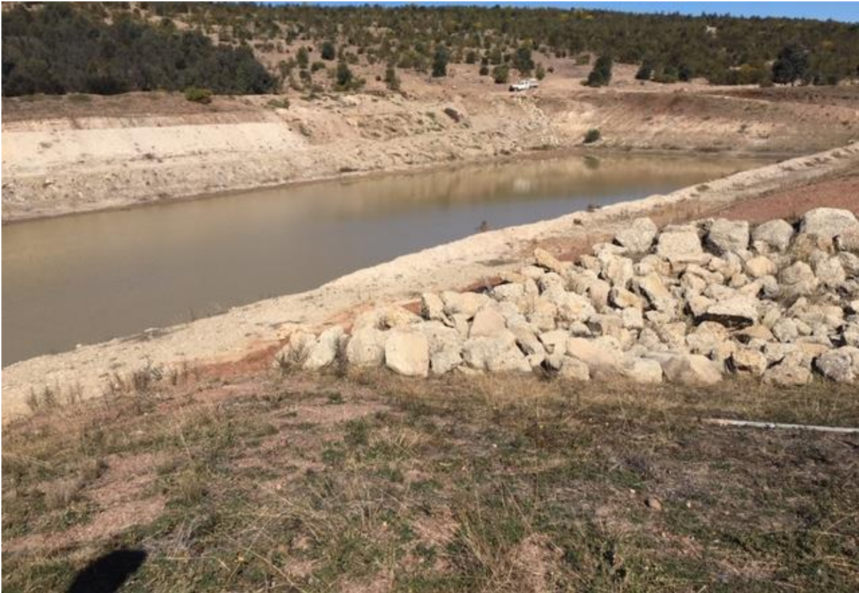
Plate 1: NOOP1 Sediment Dam with Rockfill Armoured Spillway
