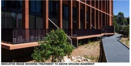
WALLS WITH SET BACK NATURAL VENTILATION TO BASEMENT SOURCE: SMART DESIGN - ARLINGTON
