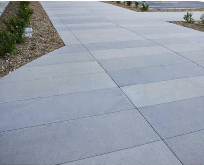
Concrete paving with saw cut
