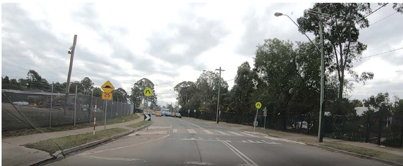
Figure 5.8: Werrington Road Pedestrian Crossing – south approach
