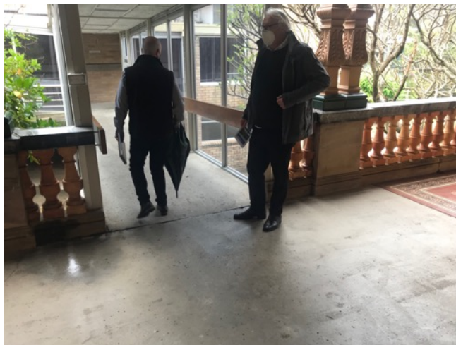
Figure 51: Verandah balustrade, handrail and concrete screed over mosaic tiles.
