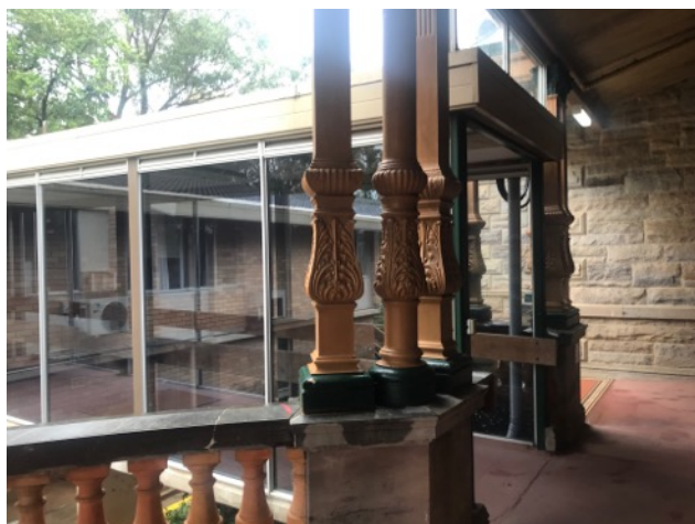
Figure 55: Verandah balustrade, handrail and concrete screed over mosaic tiles.
