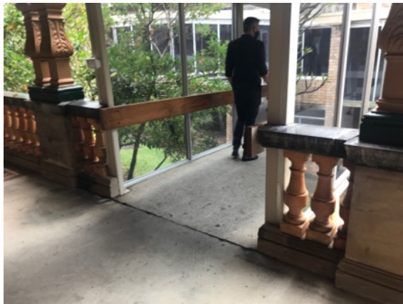
Figure 53: Verandah balustrade, handrail and concrete screed over mosaic tiles.
