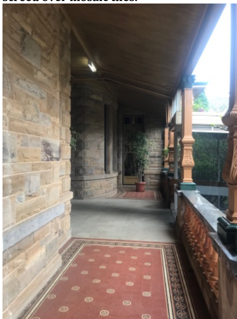
Figure 54: Verandah balustrade, handrail and concrete screed over mosaic tiles.
