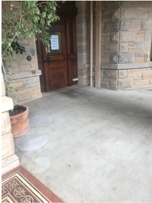
Figure 52: Verandah concrete screed over existing mosaic tiles.
