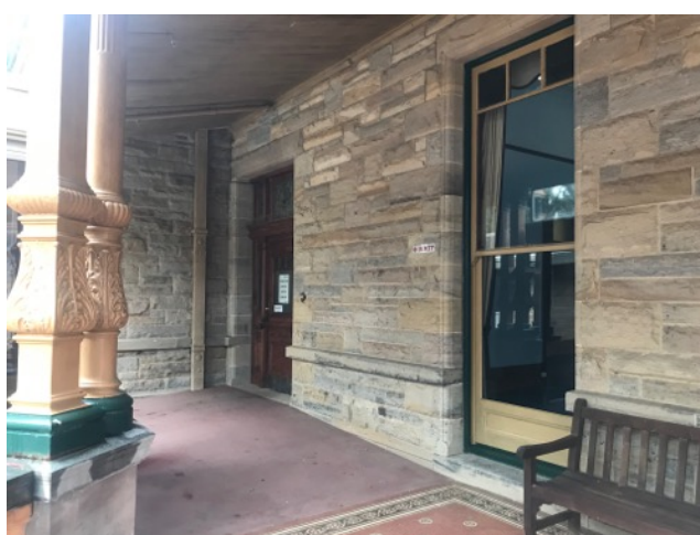
Figure 56: Verandah balustrade, handrail and concrete screed over mosaic tiles.
