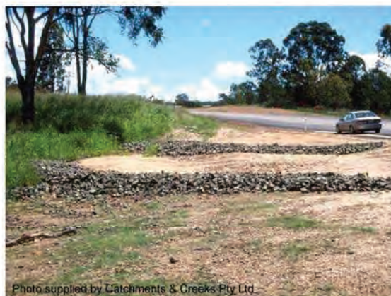
Photo 2 – Rock check dam sediment traps
