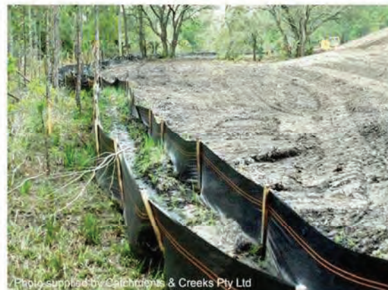
Photo 8 – Double sediment fence
