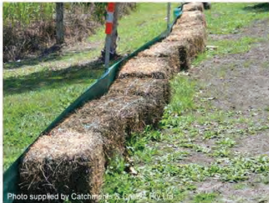
Photo 17 – Straw bales placed up-slope of the fence to separate sediment and fabric
