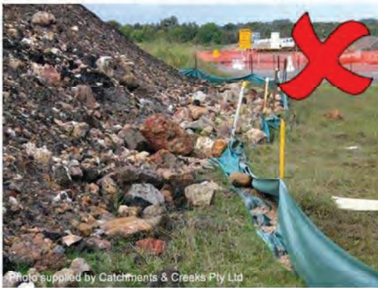
Photo 31 – Damage by shifting fill
