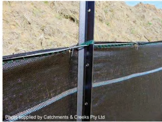
Photo 22 – Installation with top wire support
