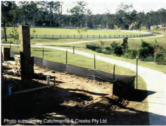
Photo 21 – Installation without backing weir/mesh
