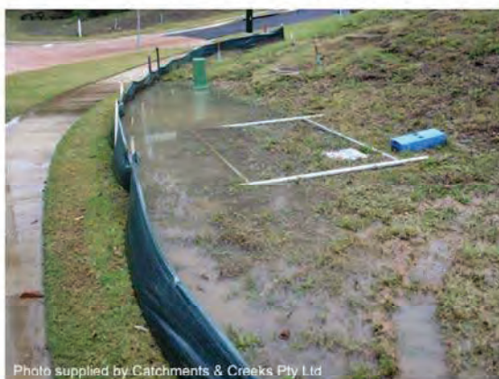
Photo 9 – Sediment fence placed along the contour
