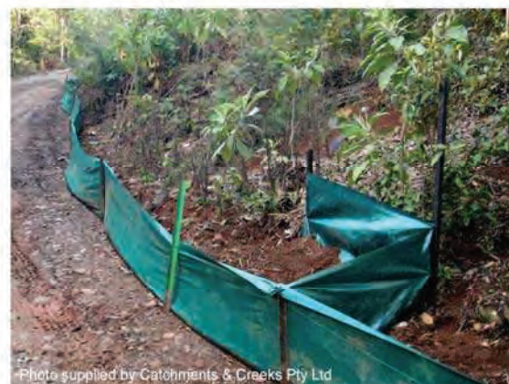
Photo 12 – Alternative design of a fence 'return'
