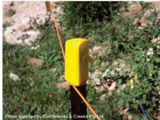
Photo 28 – Safety cap on a steel stake
