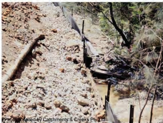
Photo 39 – Spill-through weir with up-slope aggregate filter
