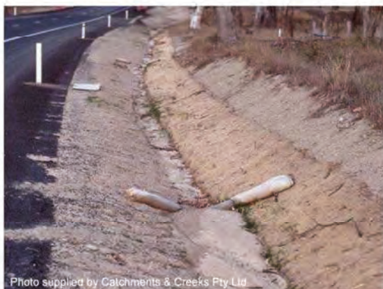
Photo 1 – Sandbag check dam sediment traps
