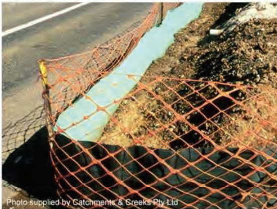
Photo 25 – Installation with safety fencing used as support
