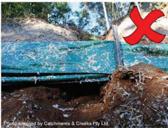
Photo 33 – Evidence of hydraulic wash-out under fence caused by poor trenching
