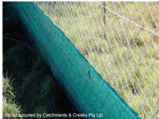
Photo 24 – Installation using fence support
