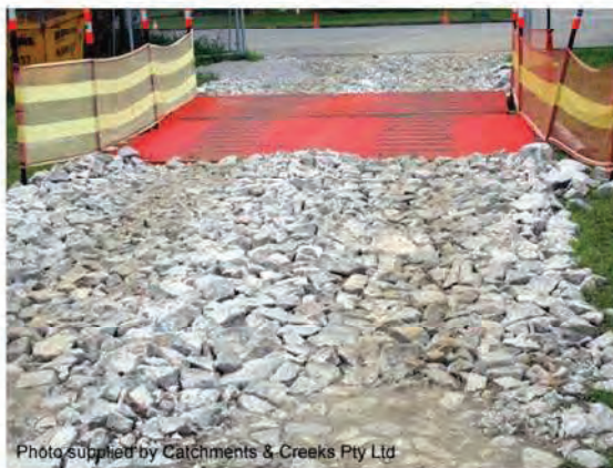
Photo 1 – Vibration grid and rock pad
