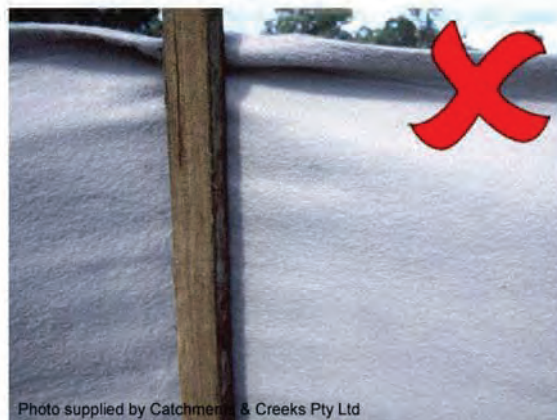
Photo 6 – Filter cloth MUST NOT be used unless used in the construction of a 'Filter Fence' adjacent to a stockpile
