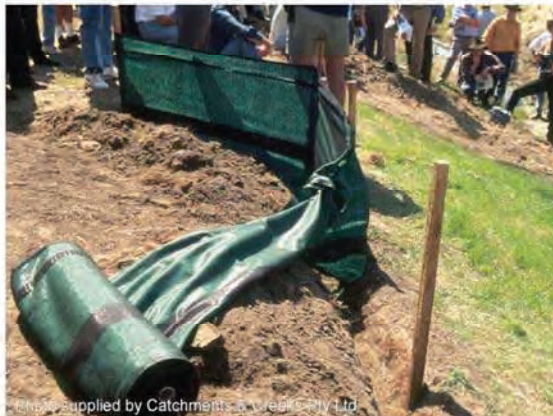
Photo 1 – Installation of a sediment fence
