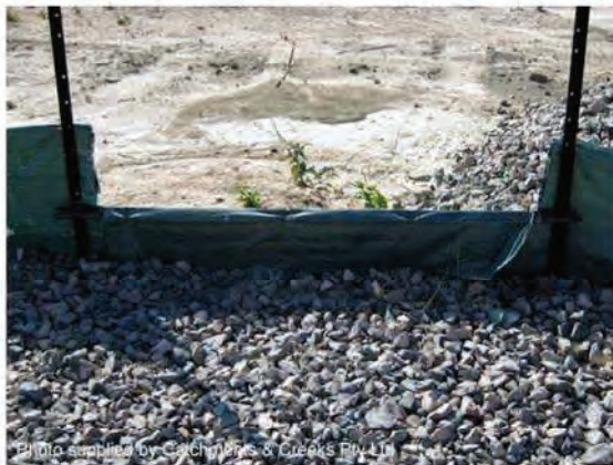
Photo 37 – Spill-through weir (down-slope side) with rock splash pad
