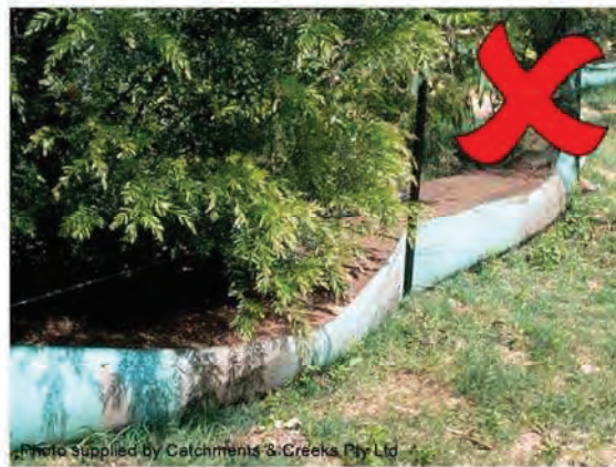
Photo 34 – Sediment not removed after storm
