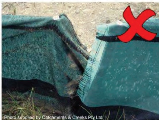
Photo 19 – Inappropriate junction
