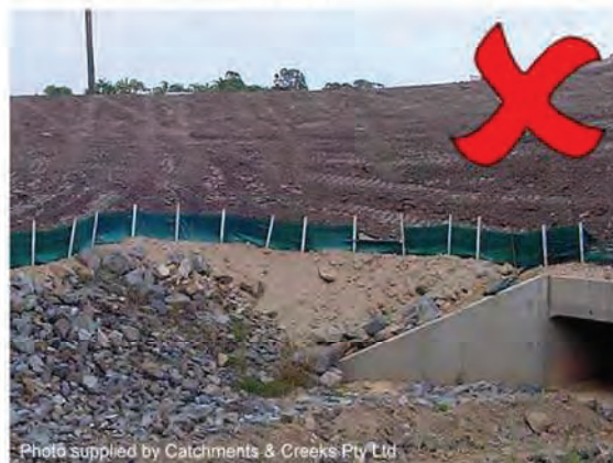
Photo 36 – Spill-through weirs must not discharge onto unstable land
