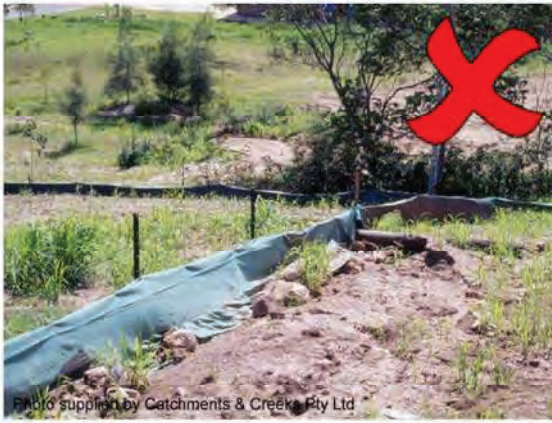
Photo 29 – Flow diversion by fence
