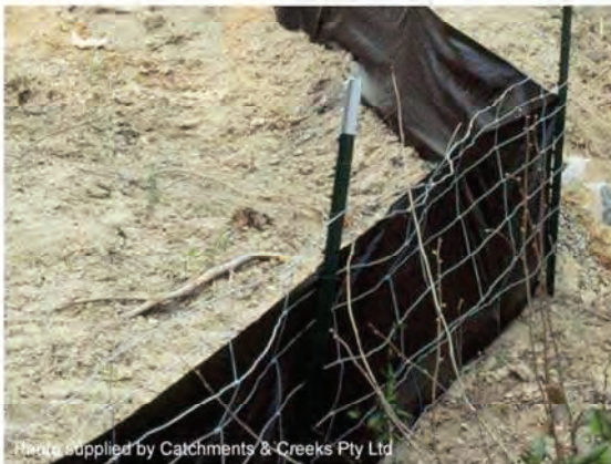
Photo 23 – Installation with weir mesh
