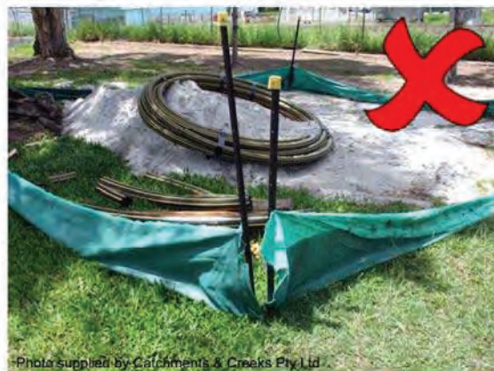
Photo 20 – Gaps in fence are not allowed
