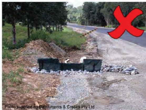
Photo 40 – Inappropriate placement of fence and installation of spill-through weir
