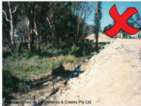
Photo 32 – Fence placed too close to fill
