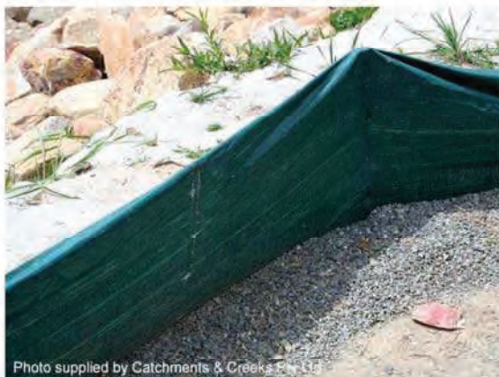
Photo 15 – Bottom of fabric buried under aggregate
