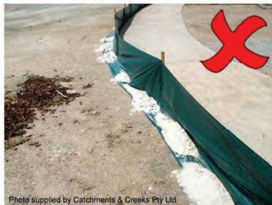
Photo 16 – Inappropriate use of sand to bury the fabric
