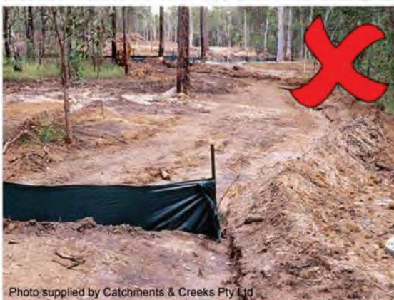
Photo 35 – Flow allowed to bypass the fence
