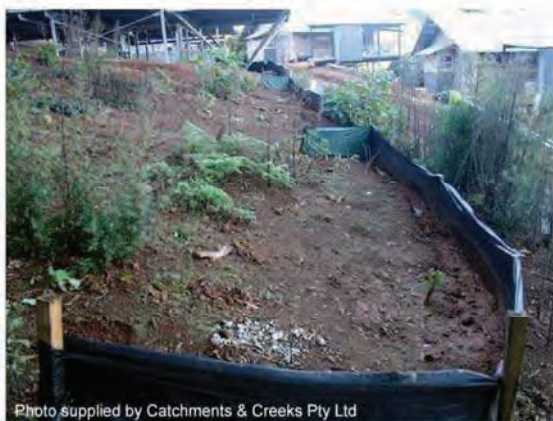
Photo 11 – Placement of fence off the contour with regular fence 'returns'
