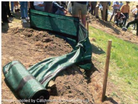
Photo 13 – Trenching the fabric
